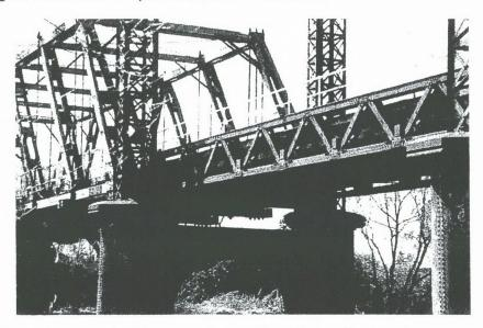
The lifting mechanism is different to that used on Hinton Bridge also over the Paterson River at Hinton, which is the junior of Dunmore Bridge by two years, and was designed by Allan's successor, EM deBurgh. The sheaves (or pulleys) at the top of the lift towers are arranged so that their axles run at right angles to the stream flow, whereas at Hinton Bridge, the arrangement of the sheaves is such that the axles parallel to the stream flow.
