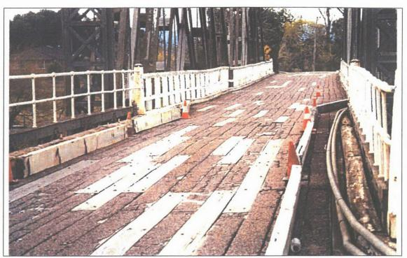
Photo 9: Timber decking to be replaced
