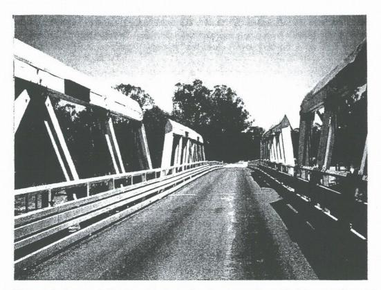
**Figure 4**: Coonamit Bridge, showing safety barrier and modified hand railing and kerb system installed. Note also appearance of SLT decking from deck level.
