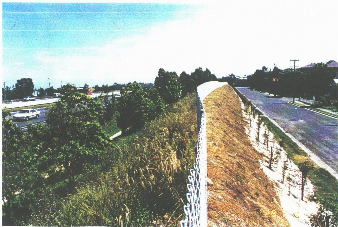
Photograph 2 Landscaped Noise Attenuation Mound Between M4 Motorway and Railway Street, Parramatta
