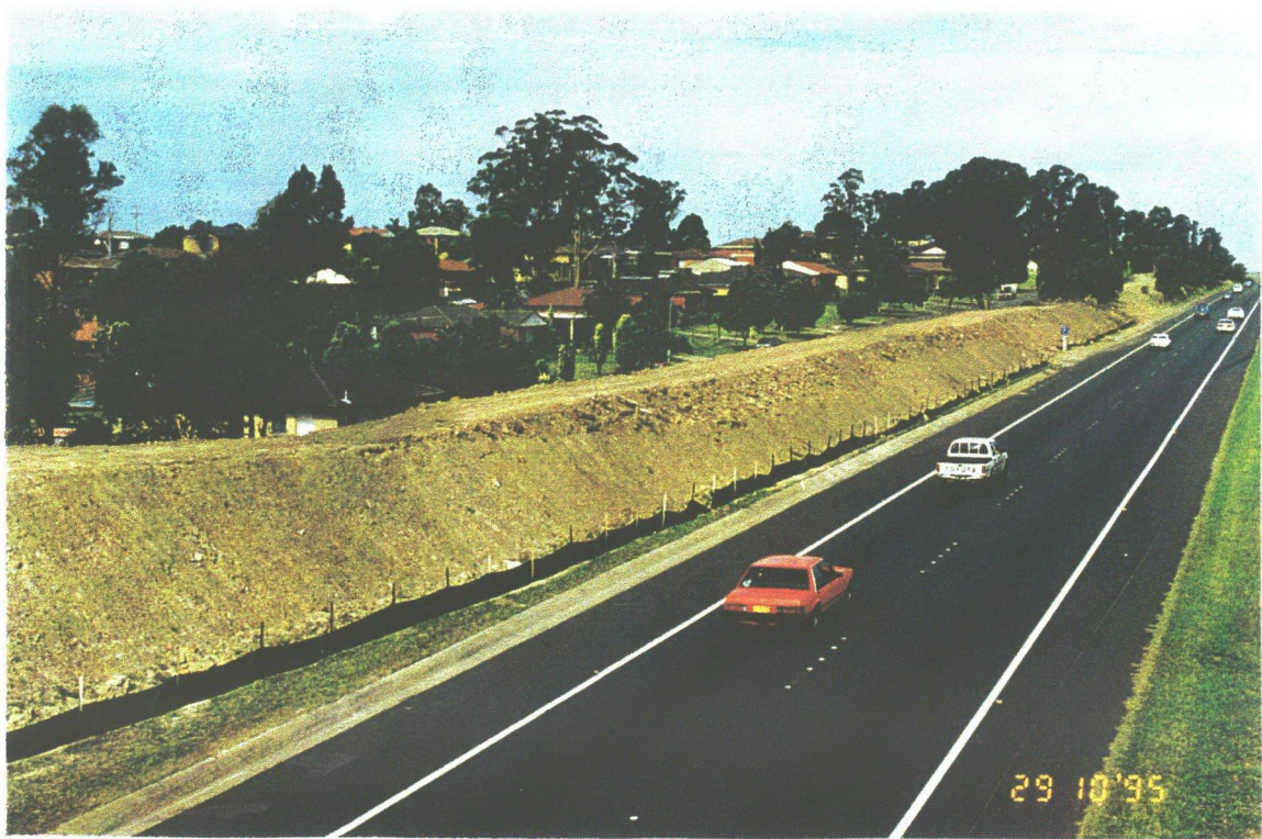
Photograph 8 Noise Attenuation Mound Under Construction Between M4 Motorway and Oliver Crescent, St Clair
