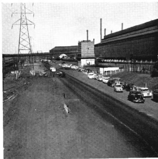
Area cleared for provision of additional two-lane carriageway in Five Islands Road.
