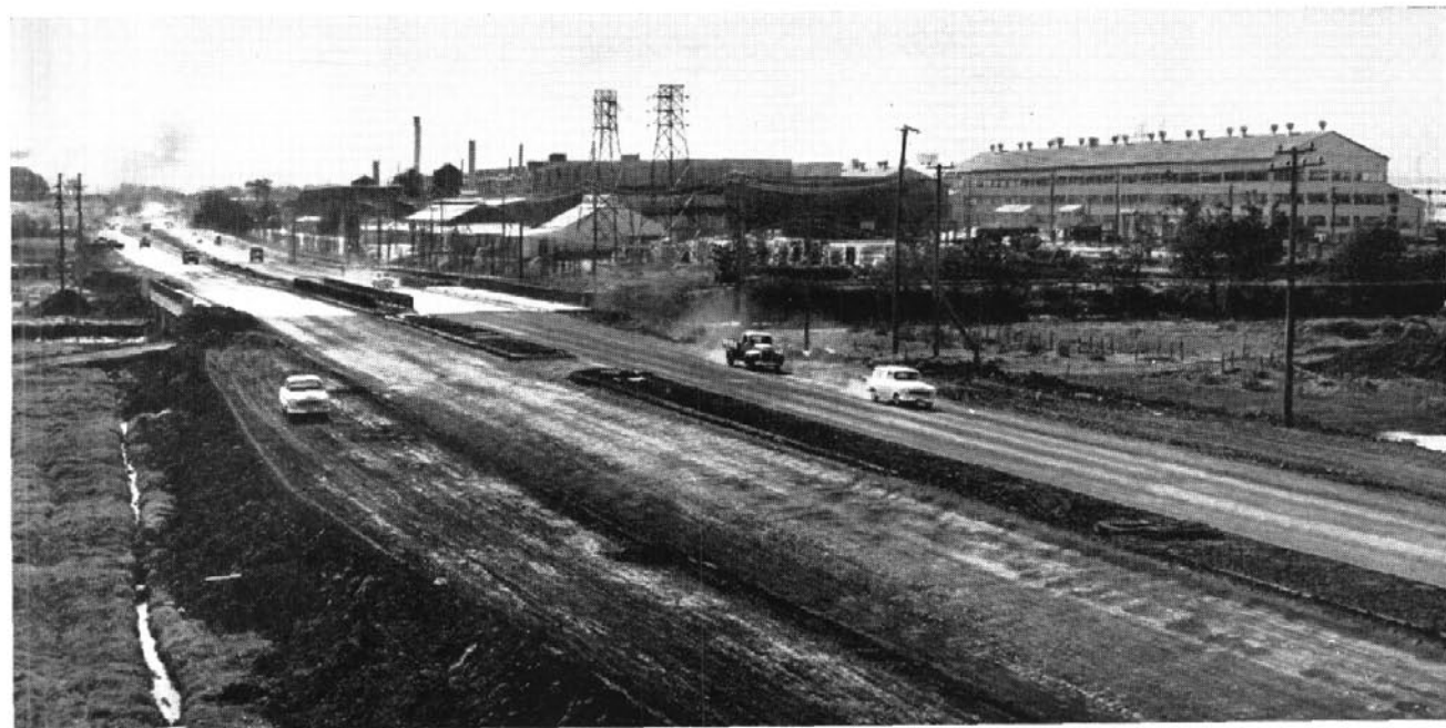
Additional two-lane carriageway under construction alongside existing carriageway in Springhill Road.
