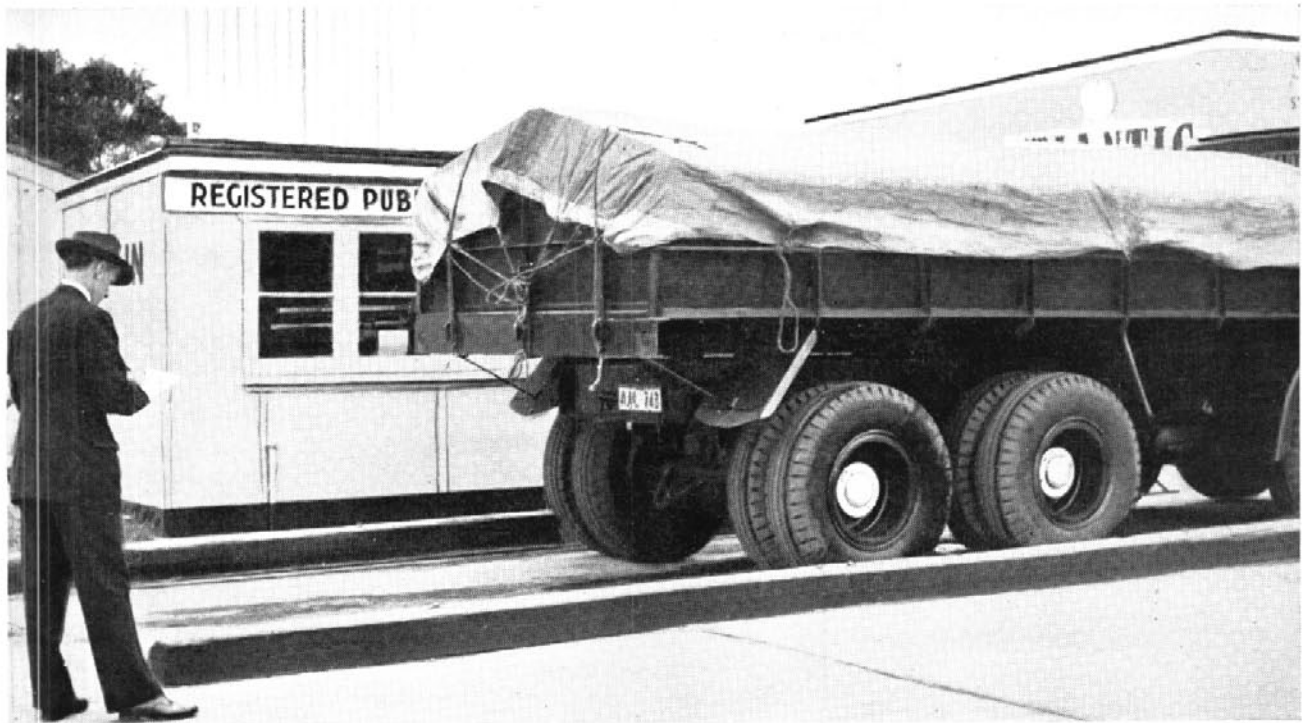
Weighing of rear axles at public weighbridge.
