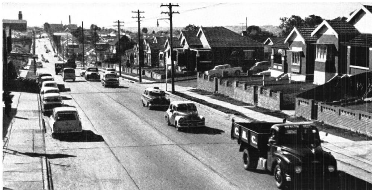
Widened cement concrete pavement in Canterbury Road looking from Quigg Street towards Victory Street. Municipality of Canterbury.
