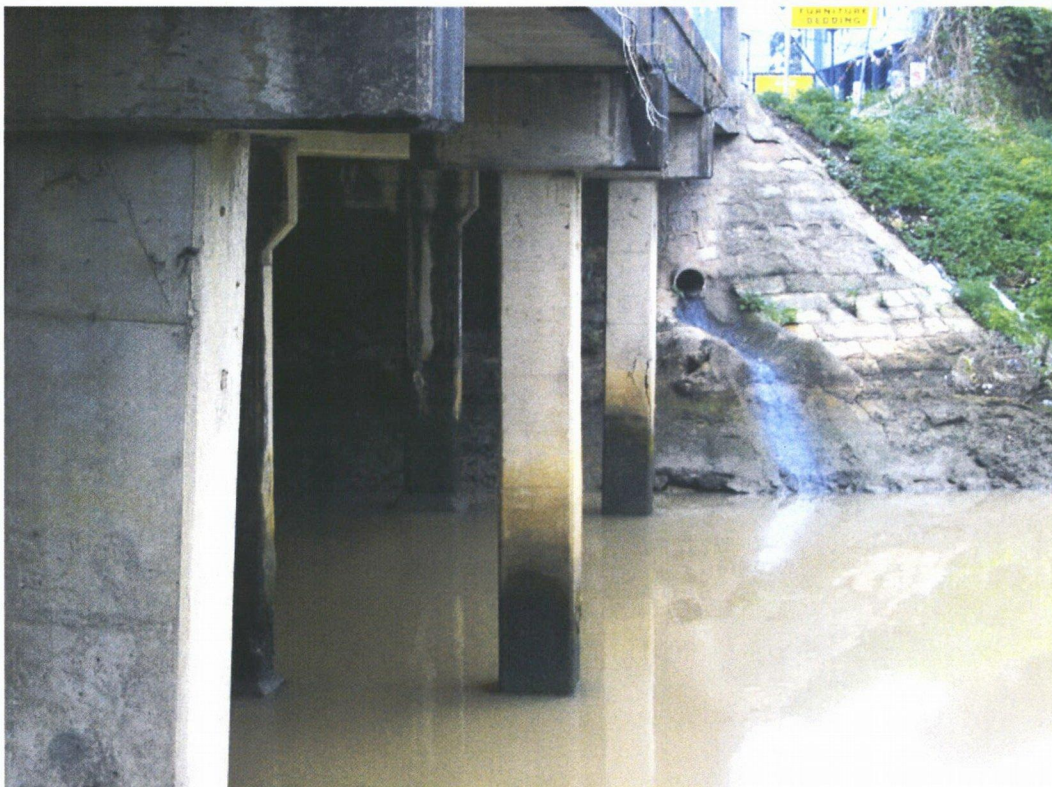
Photo 2: Drain hole on northwest abutment
