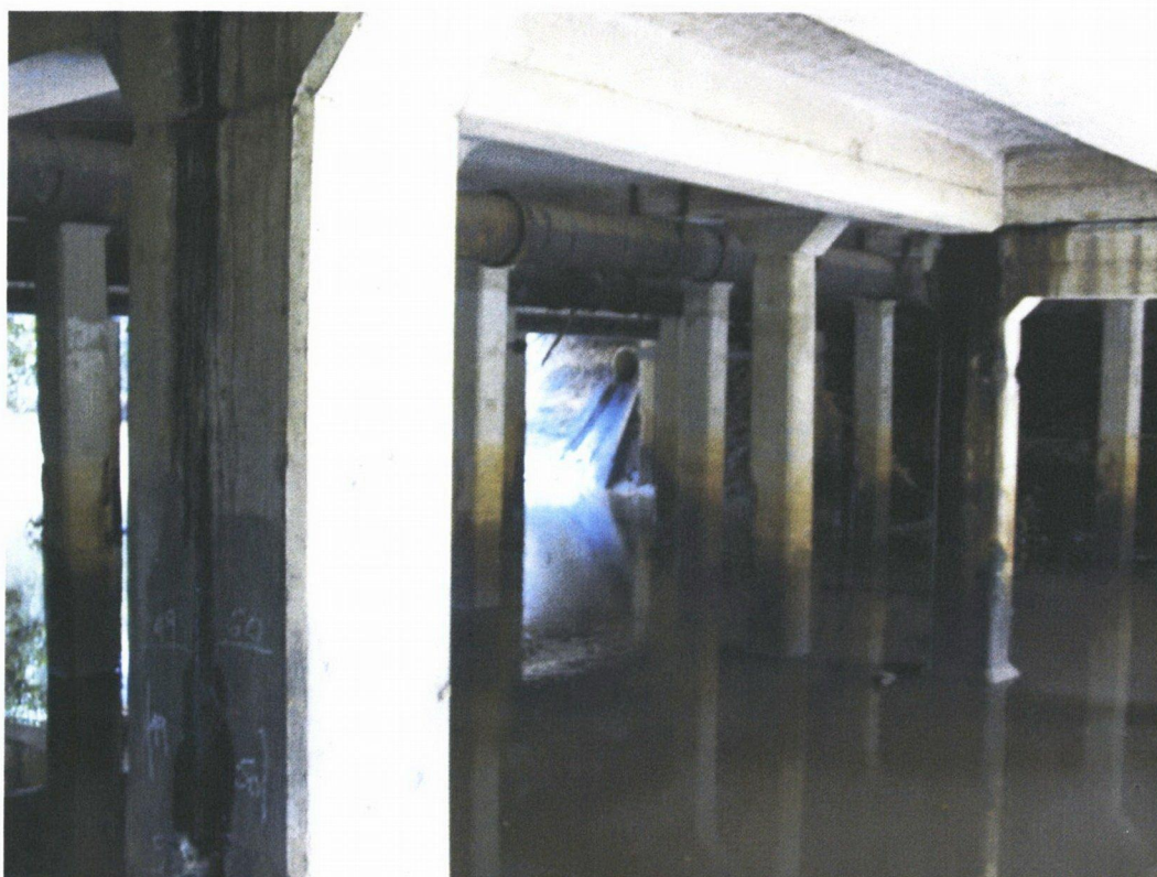
Photo 3: Underside of Bridge and drain on southwest abutment (in background)
