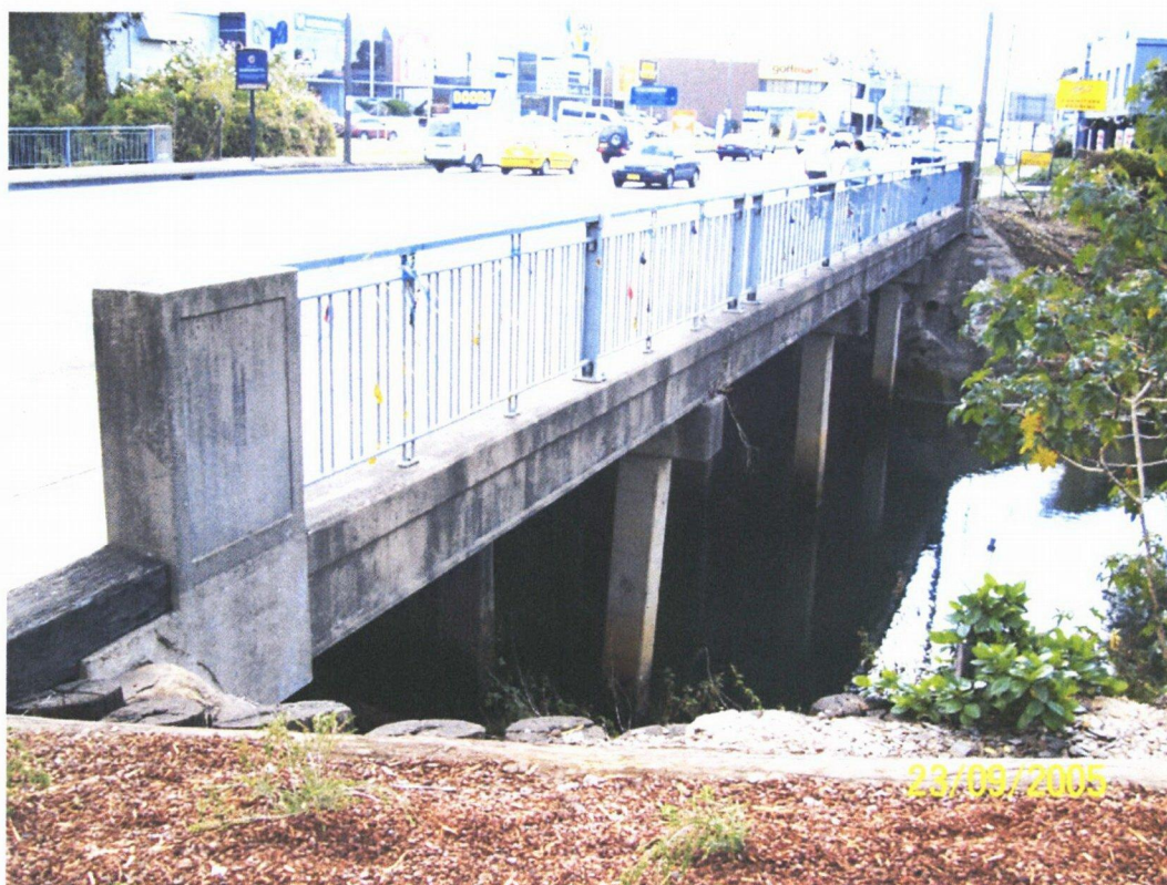
Photo 4: Appearance of Bridge to road users
