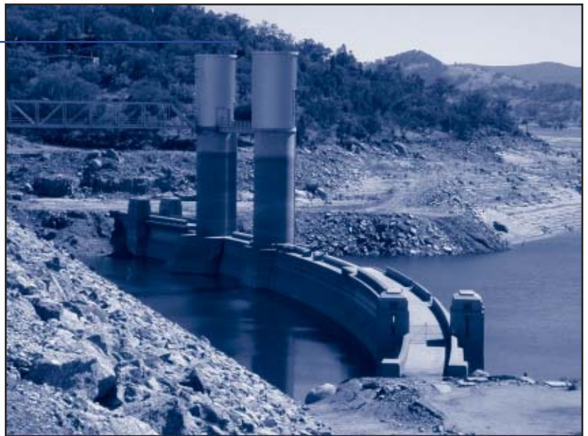
Wyangala Dam at 22% capacity, December 2002, showing the original Dam wall
