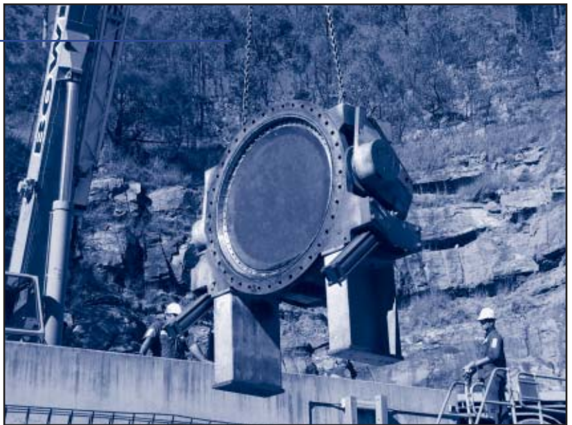
Removing the butterfly valve at Glennies Creek Dam
