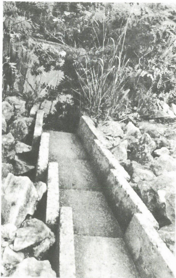
PHOTOGRAPHS 8.5/8.6: Water runoff/energy dissipator structures installed beside existing freeway
