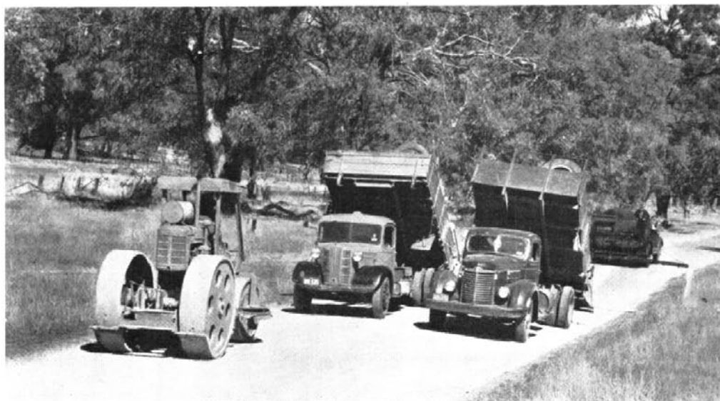
Commencement of spray run. Aggregate spreading trucks and roller in position to follow immediately spraying starts.
