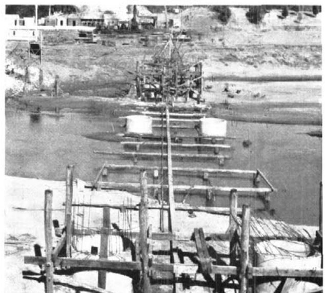
Warkworth Bridge showing work in progress on the cylinders.
