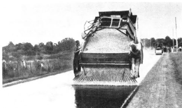
Spreading aggregate through truck tail gate and fantail spreader.
