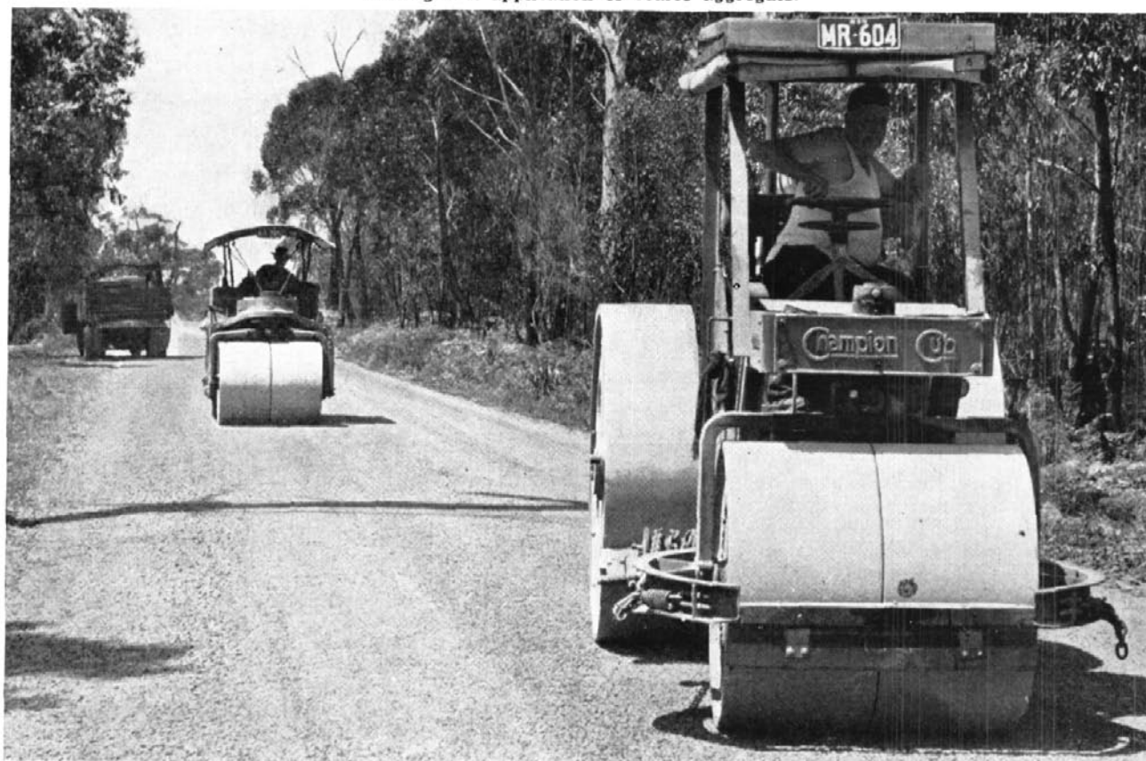
Rolling first application of coarse aggregate.
