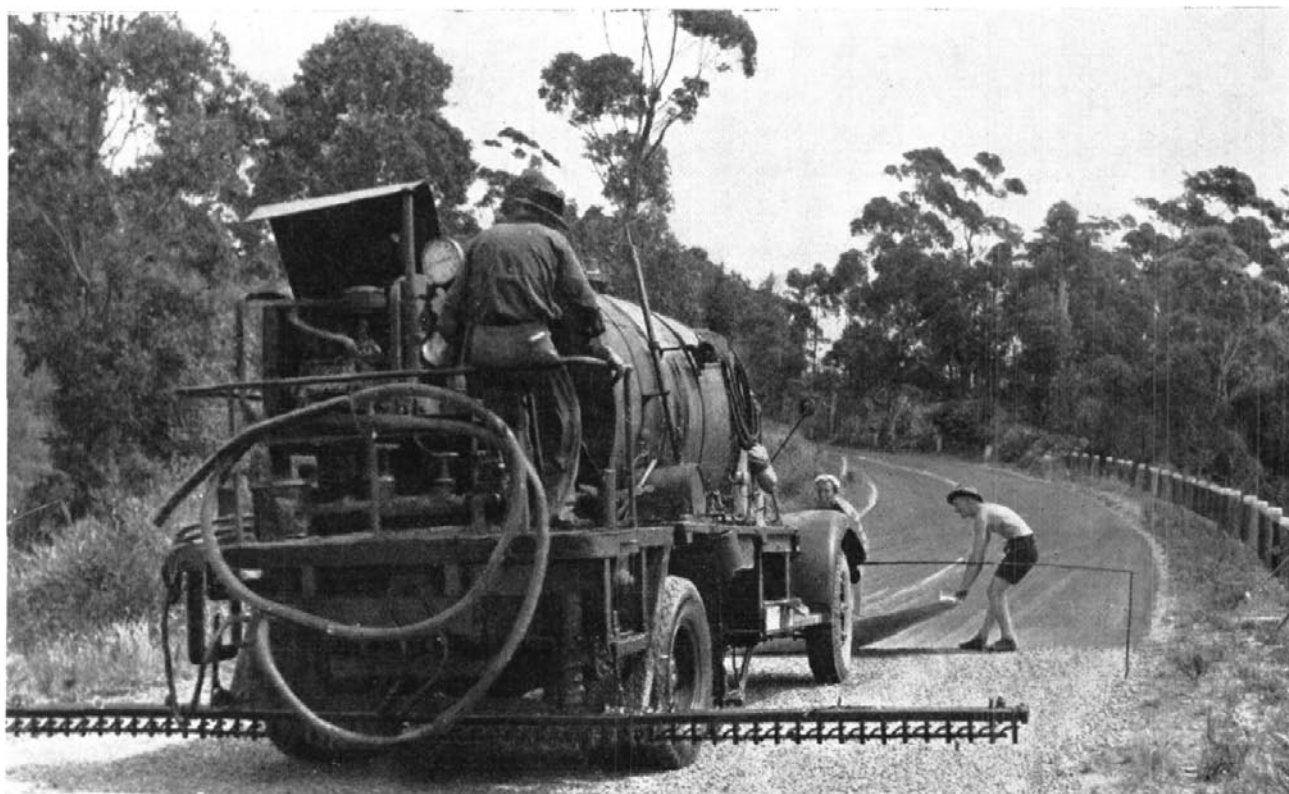
Laying paper mat for start of full width spray run. Note guide bar on sprayer.
