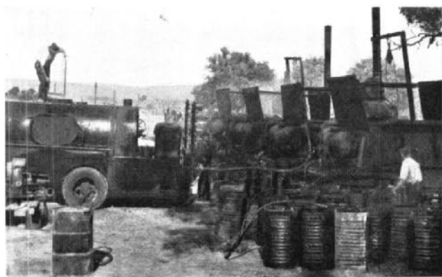
Sprayer taking delivery of hot binder from bank of oil fired kettles at Depot.
