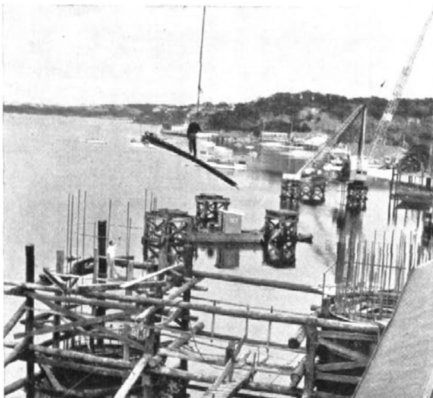
Spit Bridge Middle Harbour showing one of the piers under construction.
