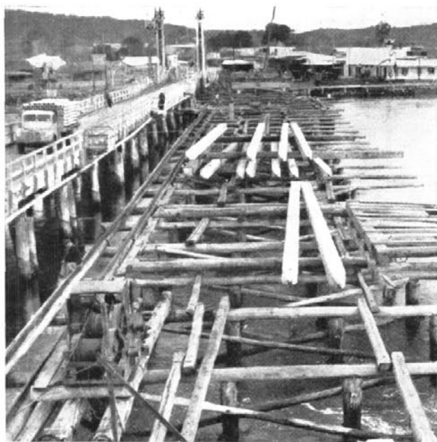
Swansea Bridge showing falsework and concrete piles for driving.
