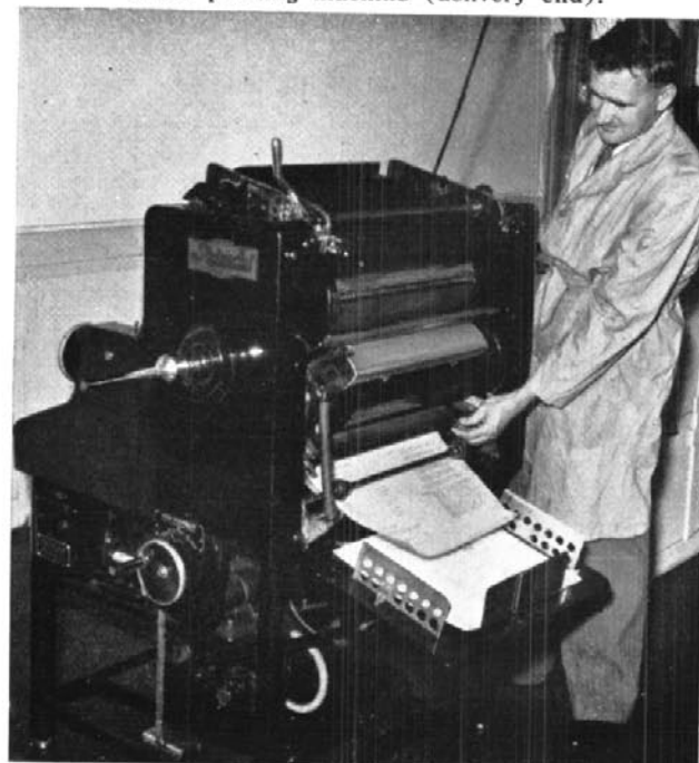
Offset printing machine (delivery end).
