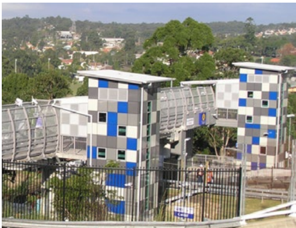
The Transport Access Program delivered a new look Cardiff Station
