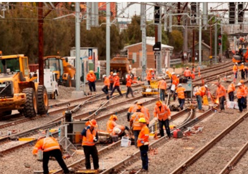
Work continues apace at Auburn Junction
