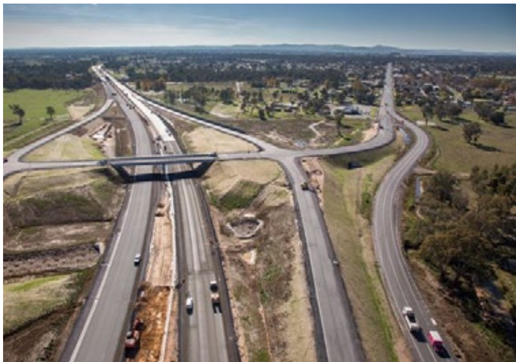
When the Holbrook bypass was completed, one of Australia's most vital roads, the Hume Highway between Sydney and Melbourne, was duplicated.
