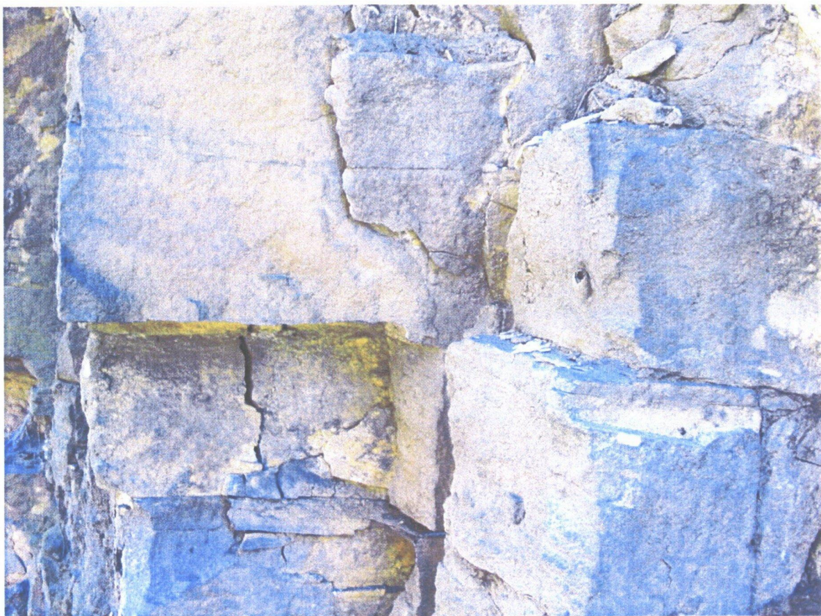
Photo 5: Cracks in cutting face causing instability
