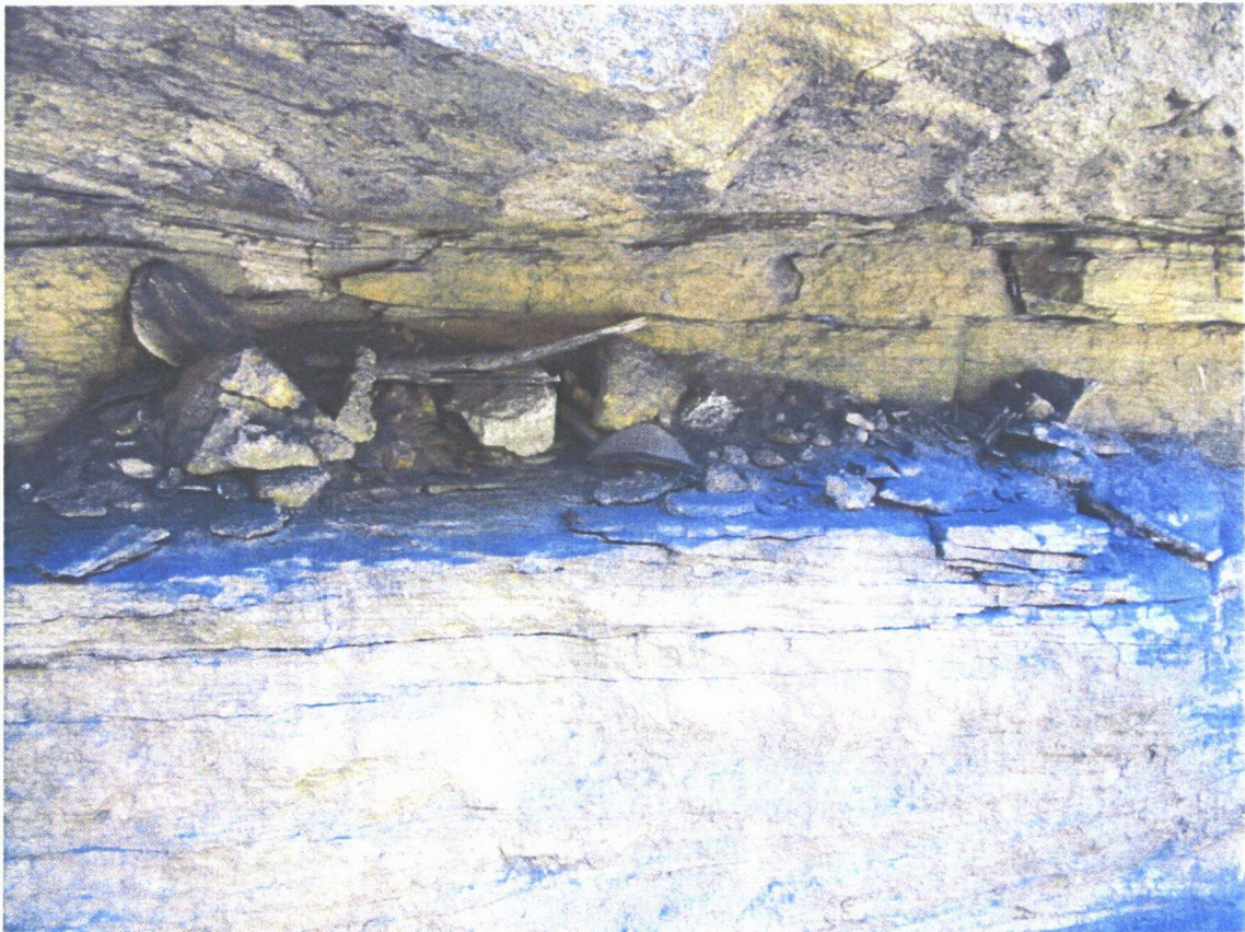
Photo 4: Soil and rock accumulations on cutting face
