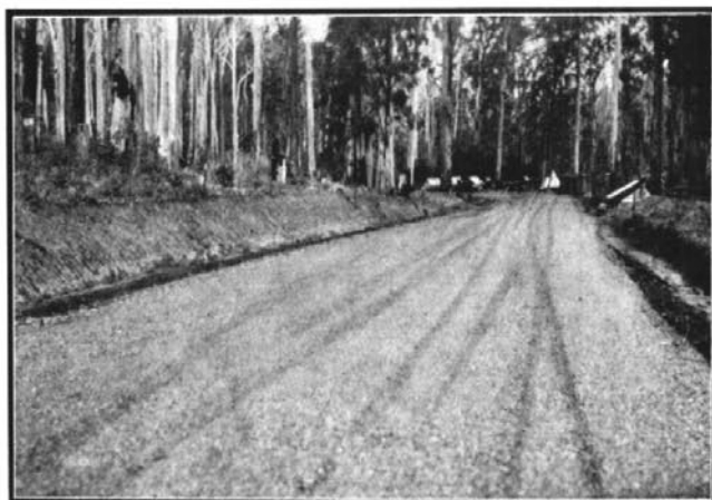
Perrot's Pinch Deviation, on the Dorriggo-Tyringham road (No. 119), near its junction with the Armidale-Grafton road (No. 120). Left, the old road. Right, portion of new deviation, 1\frac{1}{4} miles long, with water-bound macadam pavement.
