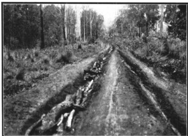
Perrot's Pinch Deviation, on the Dorriggo-Tyringham road (No. 119), near its junction with the Armidale-Grafton road (No. 120). Left, the old road. Right, portion of new deviation, 1\frac{1}{4} miles long, with water-bound macadam pavement.
