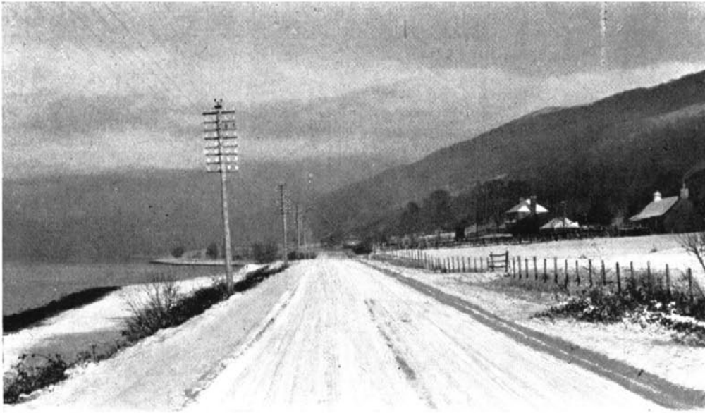
A Trunk Road near Fort William, Scotland. (Traffic not hindered by the 6 inches of snow which has fallen but a further similar fall will require clearing by plough.)
