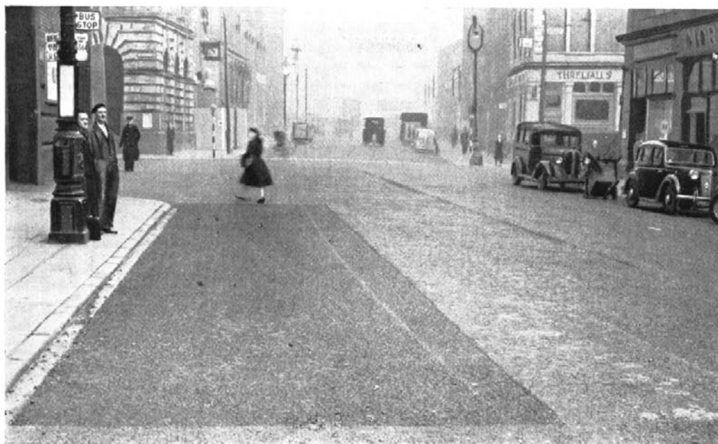
Bus Stopping Place, Whitechapel, Liverpool, specially treated to pro- duce rugose non-skid surface.
