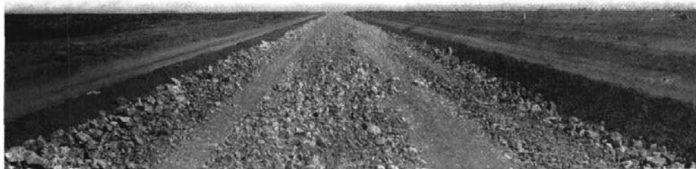
Pavement under construction using limestone gravel on raised formation, 44 miles from Bourke.
