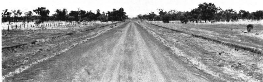
Completed Formation, approximately 100 miles from Bourke.
