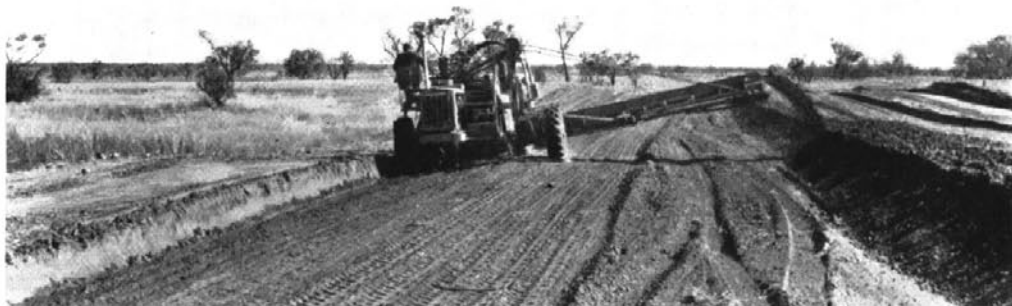
Construction of raised formation by Elevating Grader, 79 miles from Bourke.
