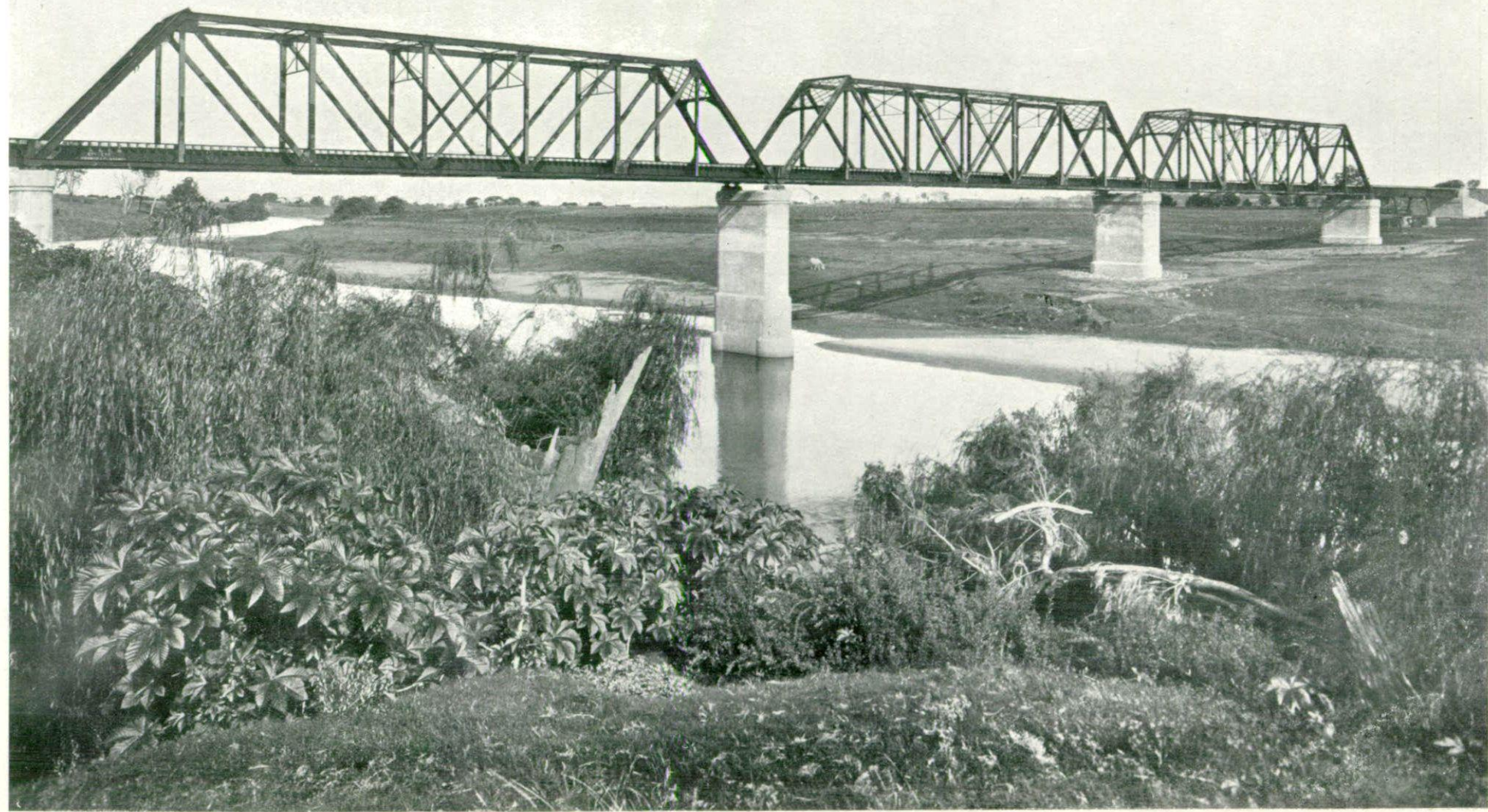
BRIDGE OVER THE HUNTER RIVER, NORTH COAST RAILWAY.
