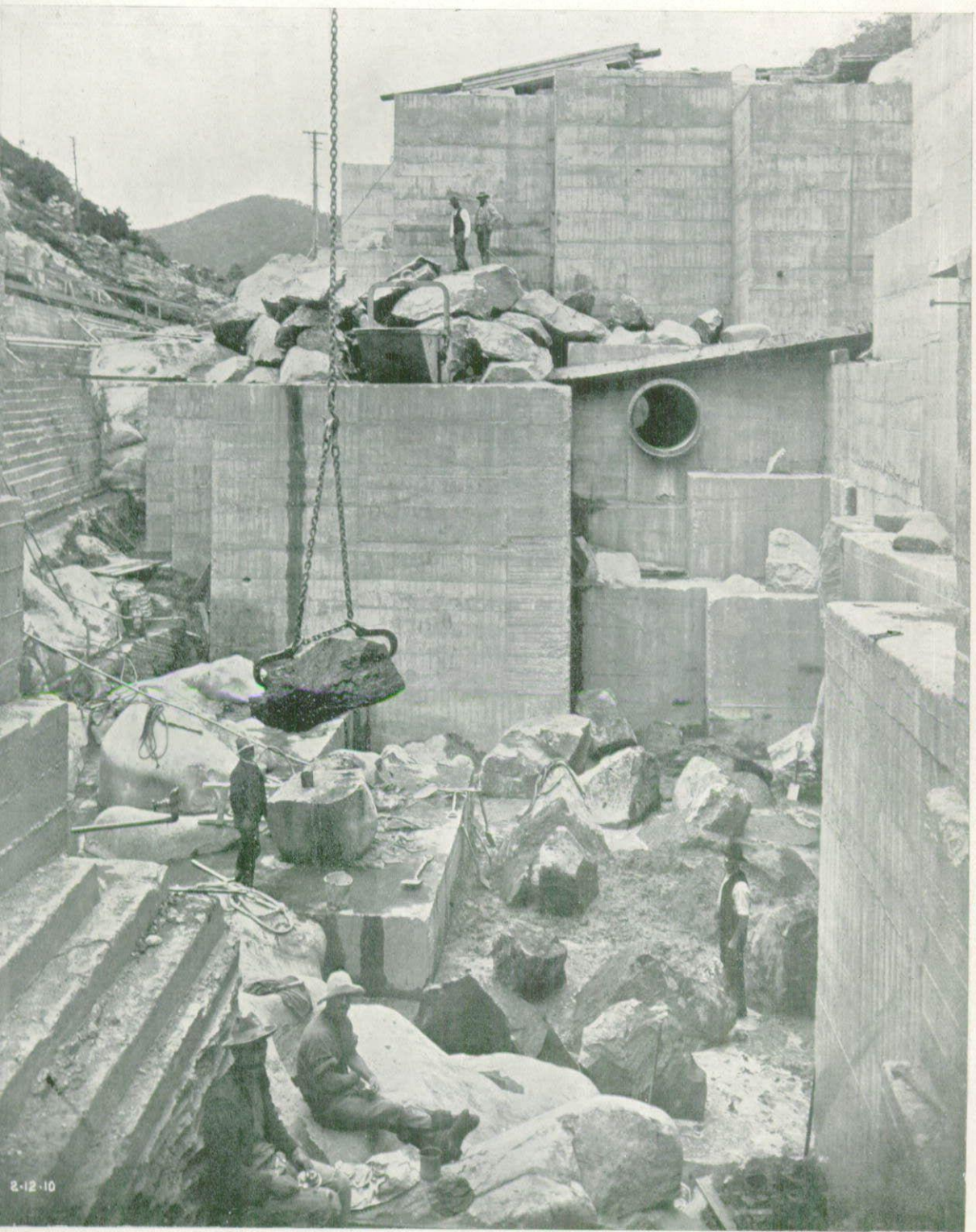
BARREN JACK DAM—UNDER CONSTRUCTION.
