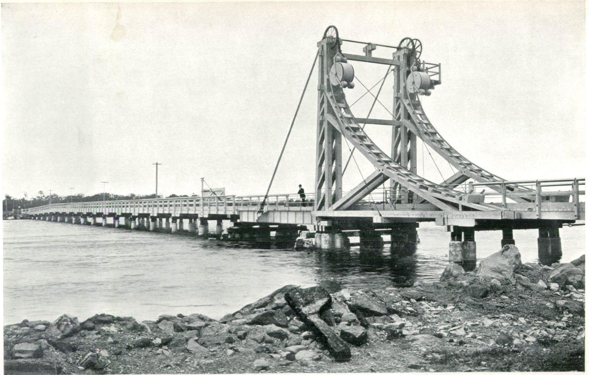
BASCULE BRIDGE, SWANSEA.
