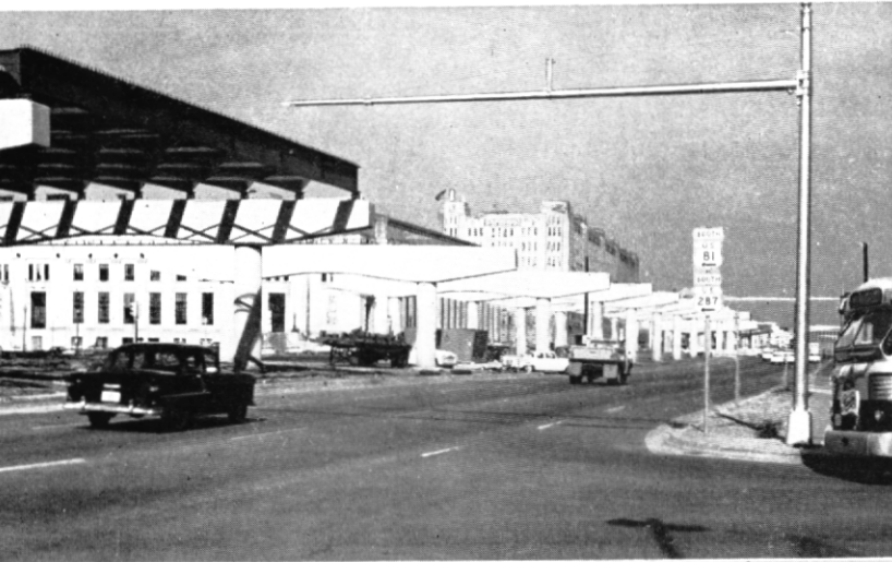
Fort Worth. Six lane elevated expressway under construction. The street will have four traffic lanes on each side of the viaduct. Full depth property acquisitions were made along one side of the street
