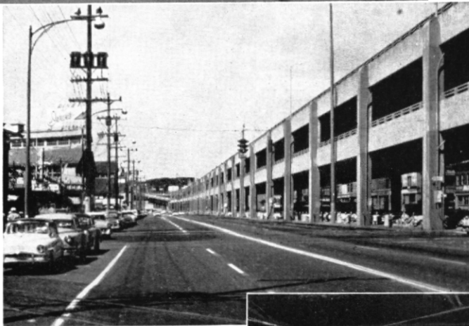
Seattle. Alaskan Way elevated expressway. On this length the space under the viaduct is used for parking, but on other lengths local traffic is carried under and parallel with the viaduct
