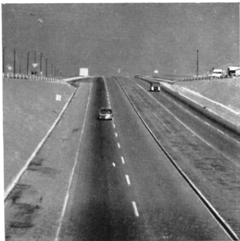
Expressway at Fort Worth. Rolling grade line giving restricted visibility
