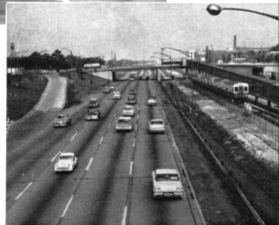
Chicago. Congress Street Expressway. Depressed construction with suburban train service operating in median.
