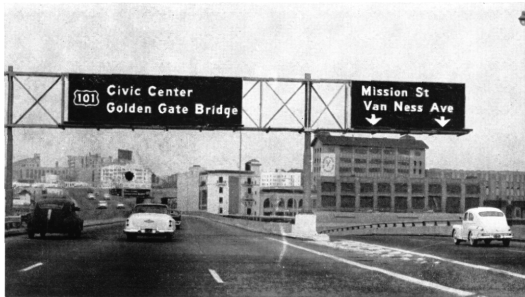
San Francisco. Typical one-deck viaduct expressway, and outlet ramp (right)
