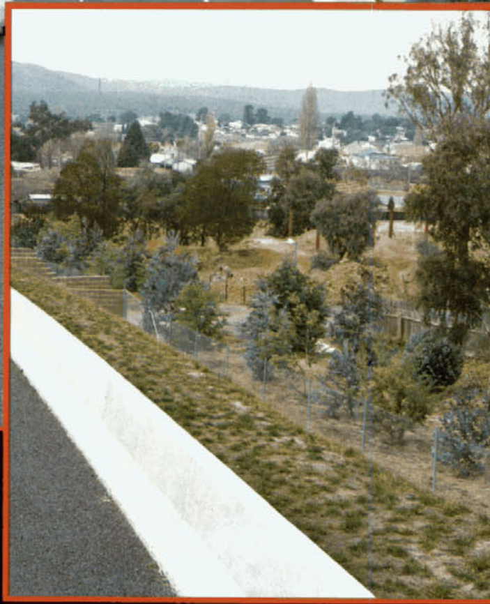
Above: Looking south towards Queanbeyan along the new dual carriageway, showing the wide shoulders and shrubs planted within the median. Right: The New Jersey crash barrier and, below the embankment, some of the 800 plants used in the Council's extensive landscaping program.
