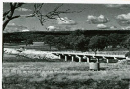
Cover: Roadworks and bridgeworks in progress near Uabry, 17 km west of Cassilis on Trunk Road No. 62.
