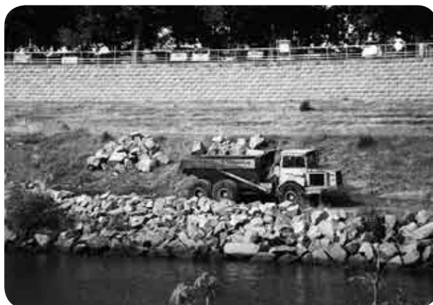
Repairs to the Maitland levee, damaged after the June 2007 floods, were completed in 2009.
