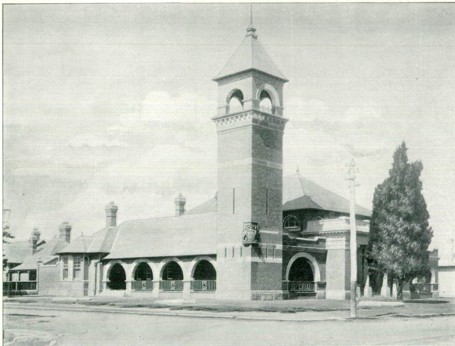
COURT HOUSE AND POLICE BUILDINGS, PARRAMATTA.
