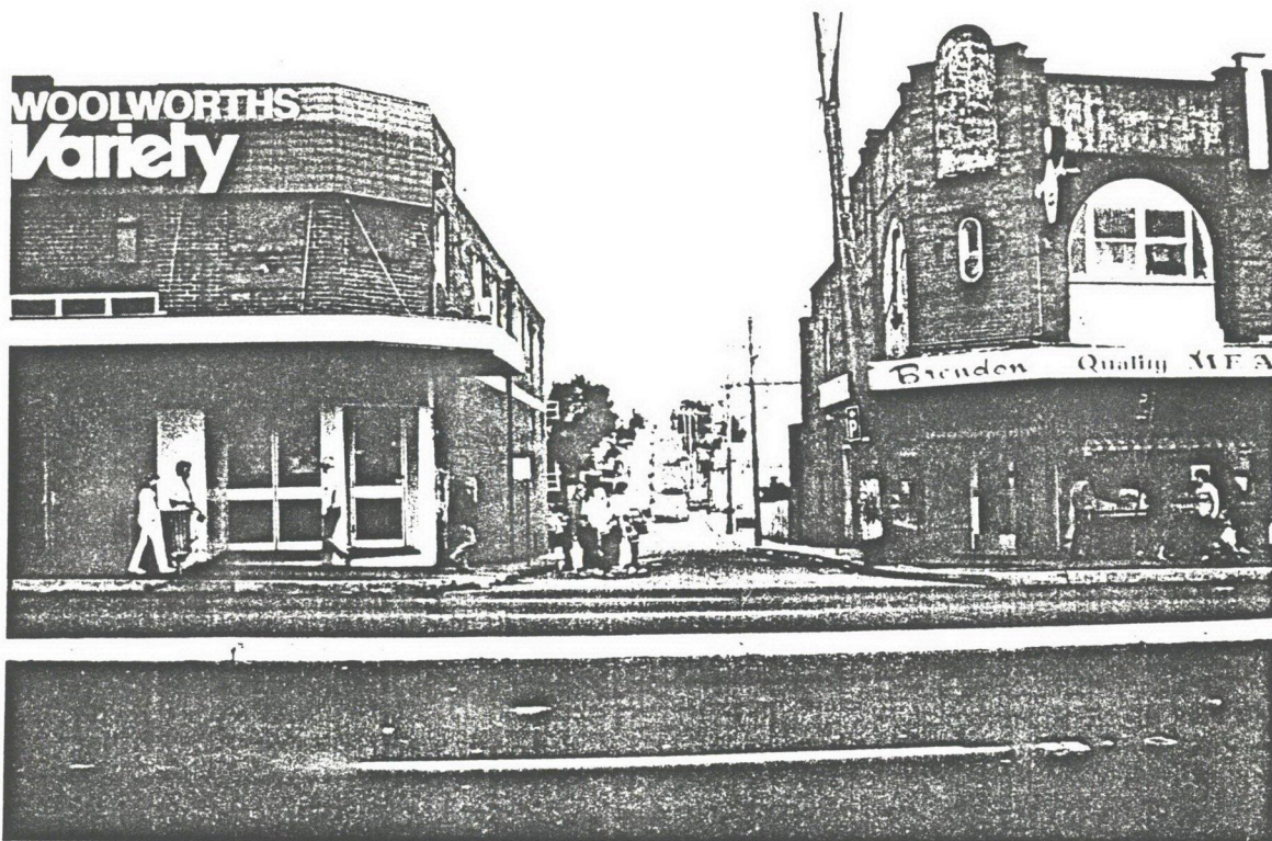
PLATE 5.4 TRAFFIC MANAGEMENT. VIEW OF HAY STREET SHOWING NARROW ONE-WAY ACCESS AND CROWDED ON-STREET PARKING.
