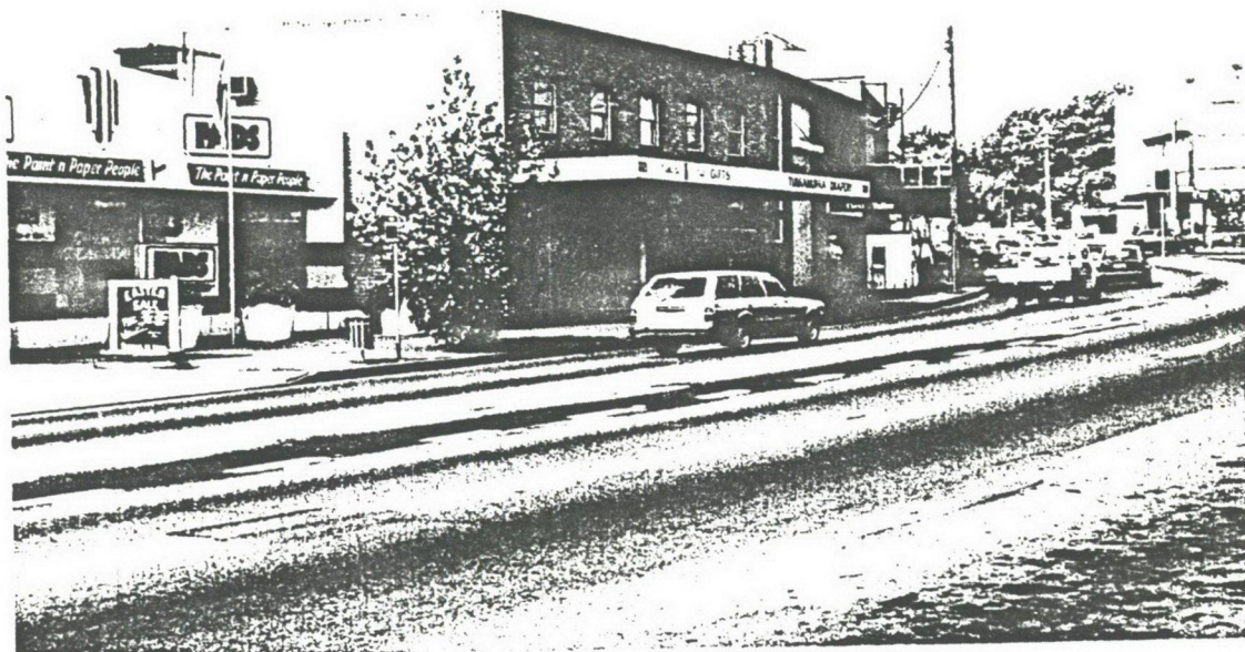
PLATE 4.4 ROAD ALIGNMENT. TURRAMURRA SHOPPING CENTRE. THE ALIGNMENT OF THE ROAD AND THE PROXIMITY OF VEHICLES TO THE KERB AND AWNINGS ARE CLAIMED TO BE RESPONSIBLE FOR A NUMBER OF RECENT ACCIDENTS, WHERE VEHICLES MOUNTED THE KERB AND CAUSED EXTENSIVE DAMAGE TO PROPERTY.
