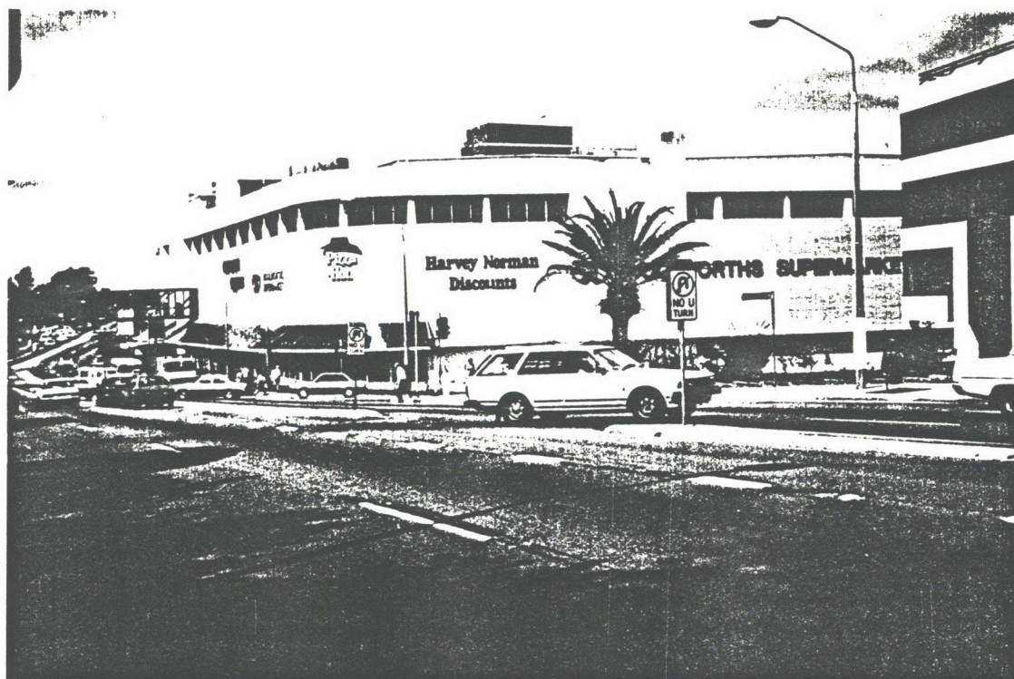
PLATE 3.7 GORDON CENTRE AND THE OVERHEAD BRIDGE.
