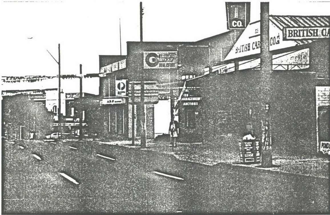
PLATE 6.3 AREA 4. AREA 4 - THE NORTH EASTERN CORNER OF THE HUME HIGHWAY / THE BOULEVARDE INTERSECTION.
