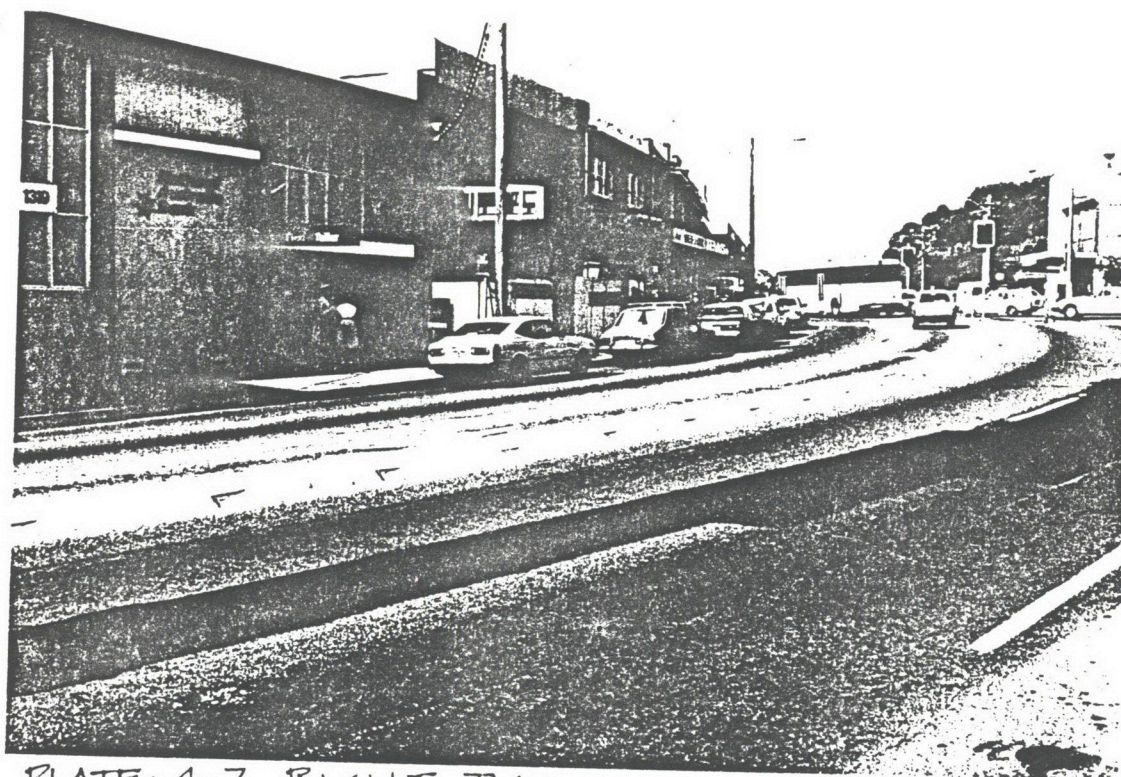
PLATE 4.7 RIGHT TURNING LANE. PACIFIC HIGHWAY, TURRAMURRA, SHOWING RIGHT HAND TURNING LANE INTO KISSING POINT ROAD.
