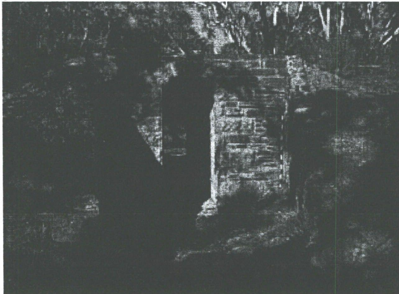
Figure 2.7: Culvert 5, view of west face. Arch height 2.54m and width 1.04m.
