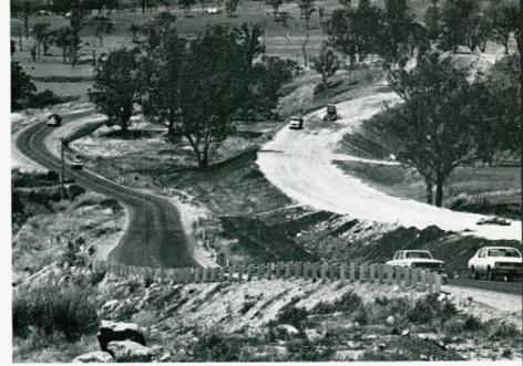
(Above): Reconstruction on the New England Highway, 3.5 km south of Muswellbrook, where this winding section will be eliminated on completion of a new section on an improved alignment and grading.
