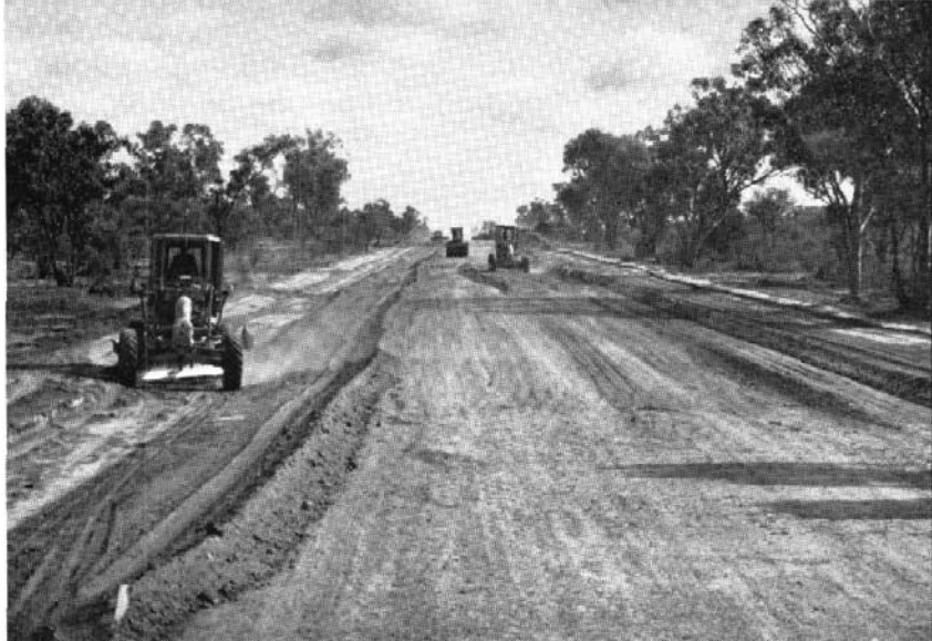
Construction work in progress on State Highway No. 7 about 61 miles north of Nyngan
