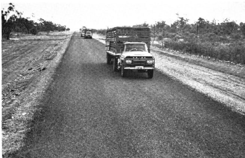
Reconstructed section 46 miles south of Bourke
