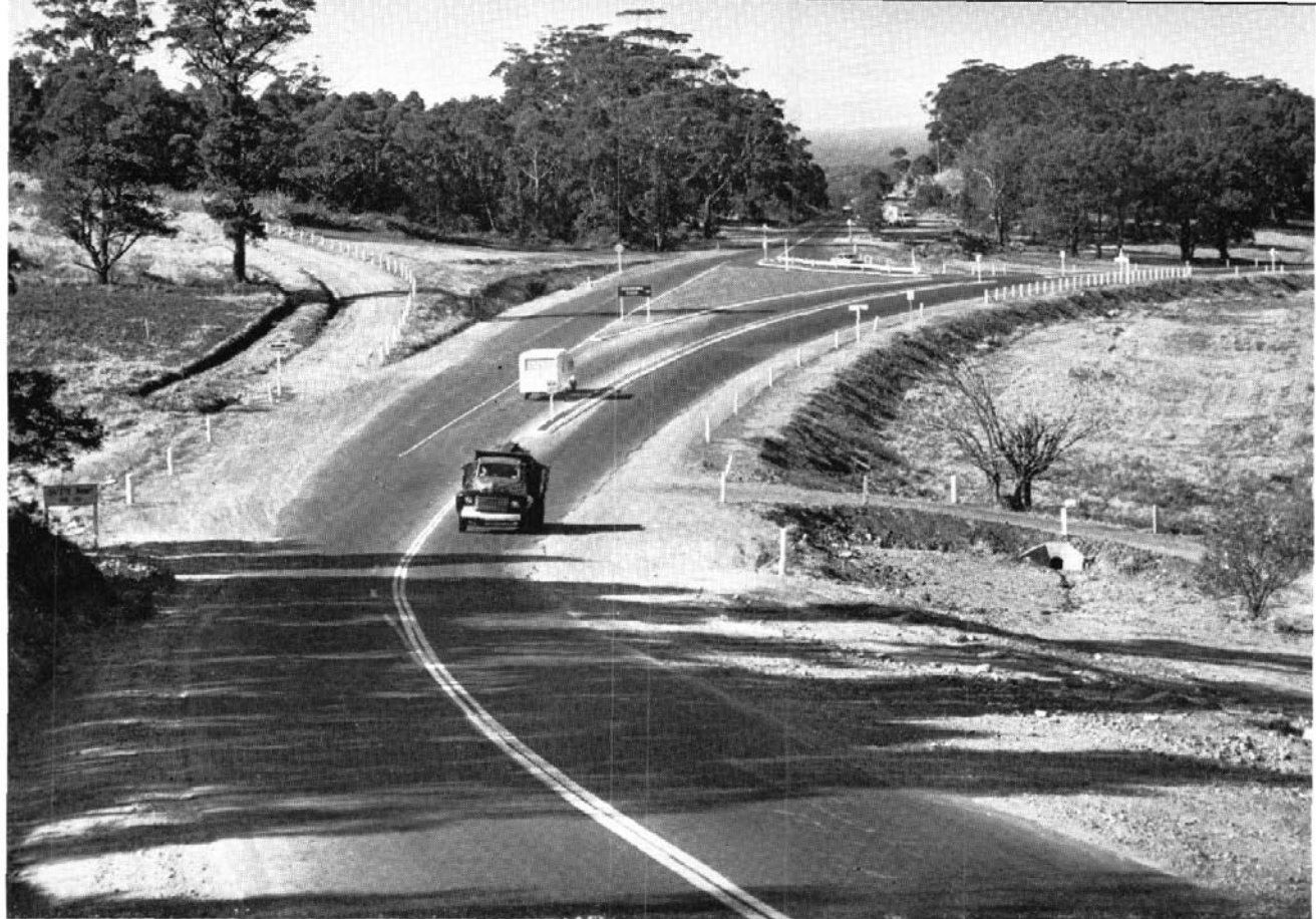
Channelised intersection at the junction of Mount Ousley Road and the Link Road
