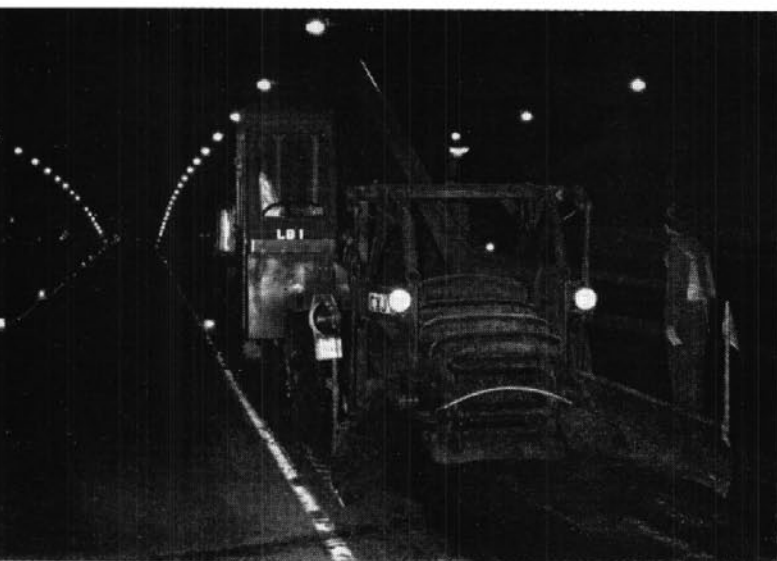
↕ The belt loader gathering the surplus material and loading on to the following truck
