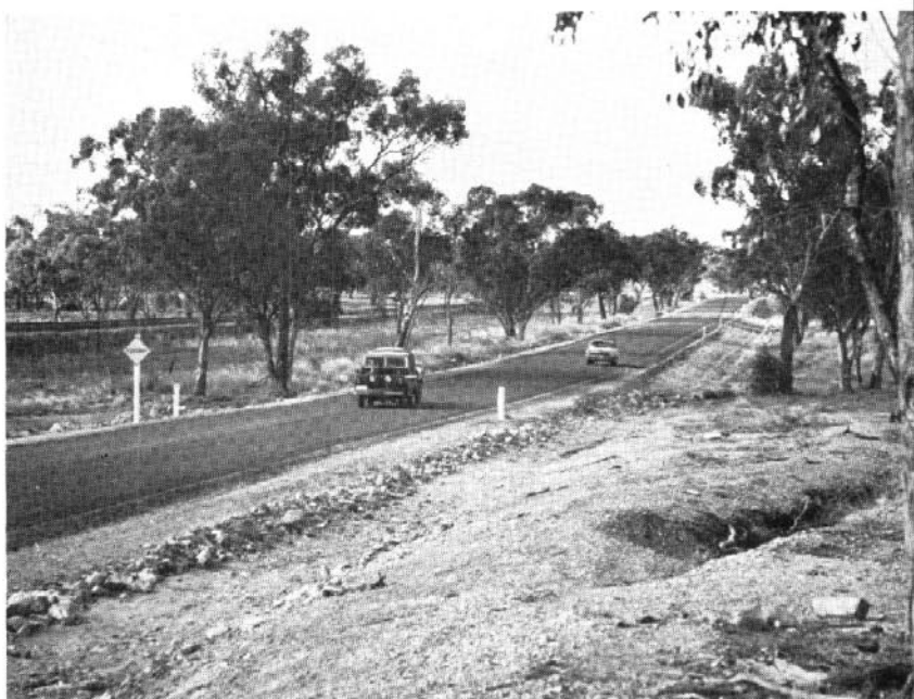
Reconstructed section of Mitchell Highway about 36 miles north of Nyngan
