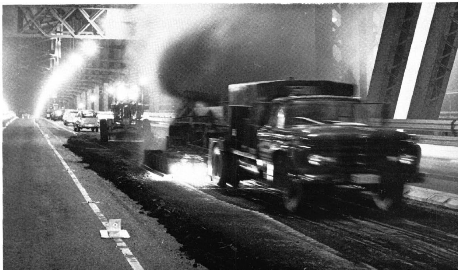
The heating unit being followed by a grader
