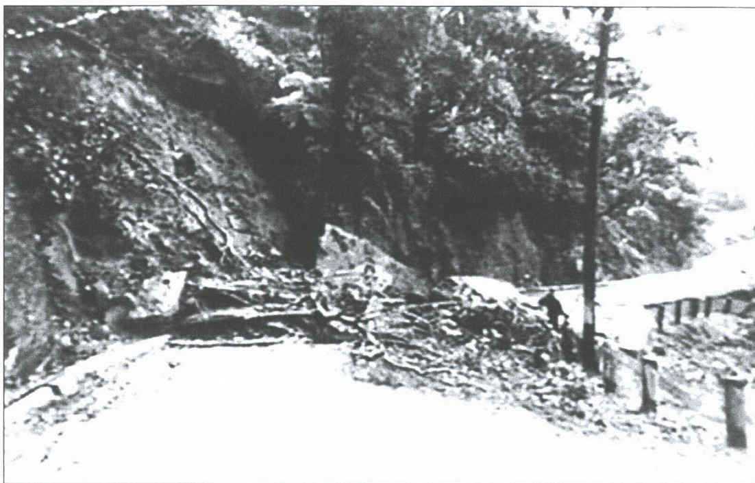
Plate 9.1: July 1949 Landslide (Source: Wollongong City Library File No. P04\P04167)
