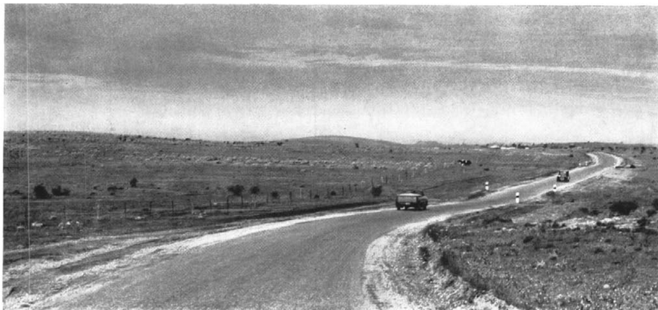
A view of the Broken Hill-Silverton-road after construction.
