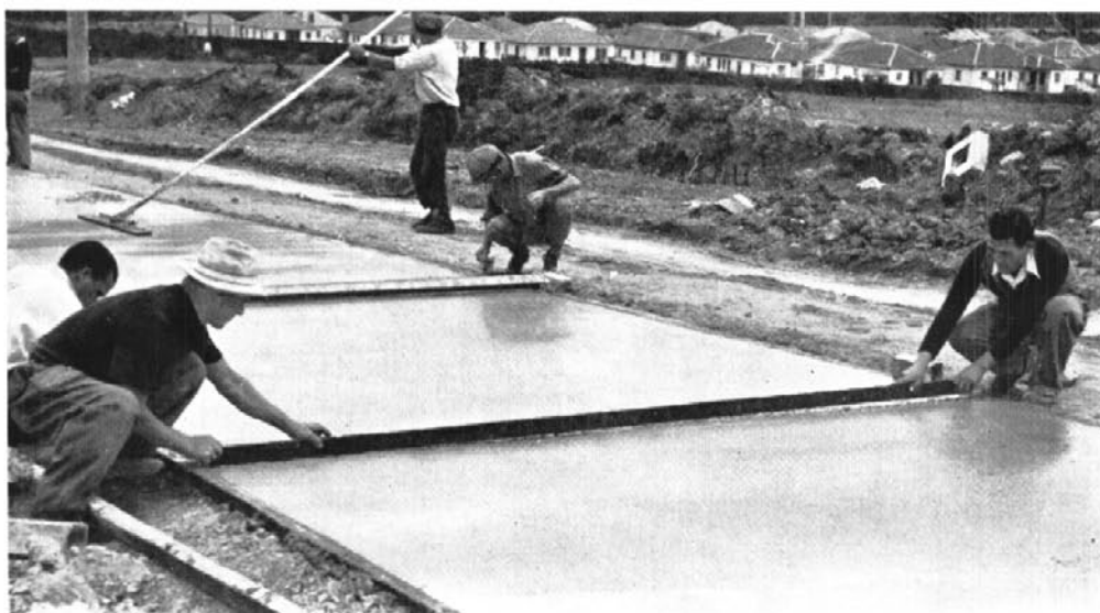
Substituting timber strip for "T" Iron.
