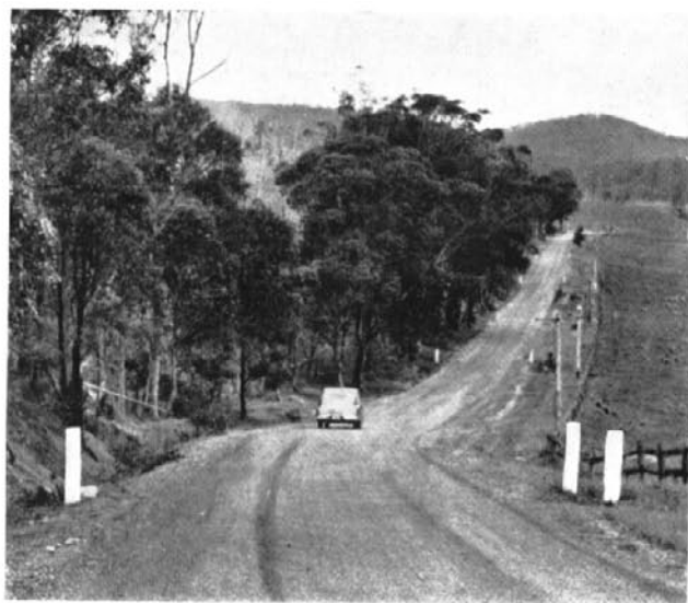
Section of completed work, Main Road No. 220, Shire of Kearsley.
