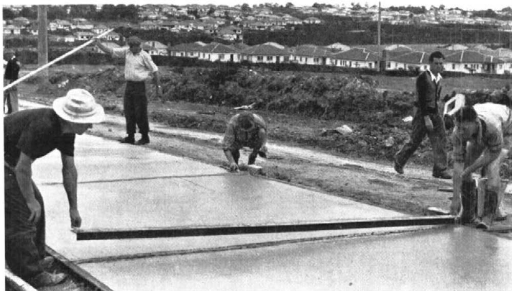
Withdrawing "T" Iron.
