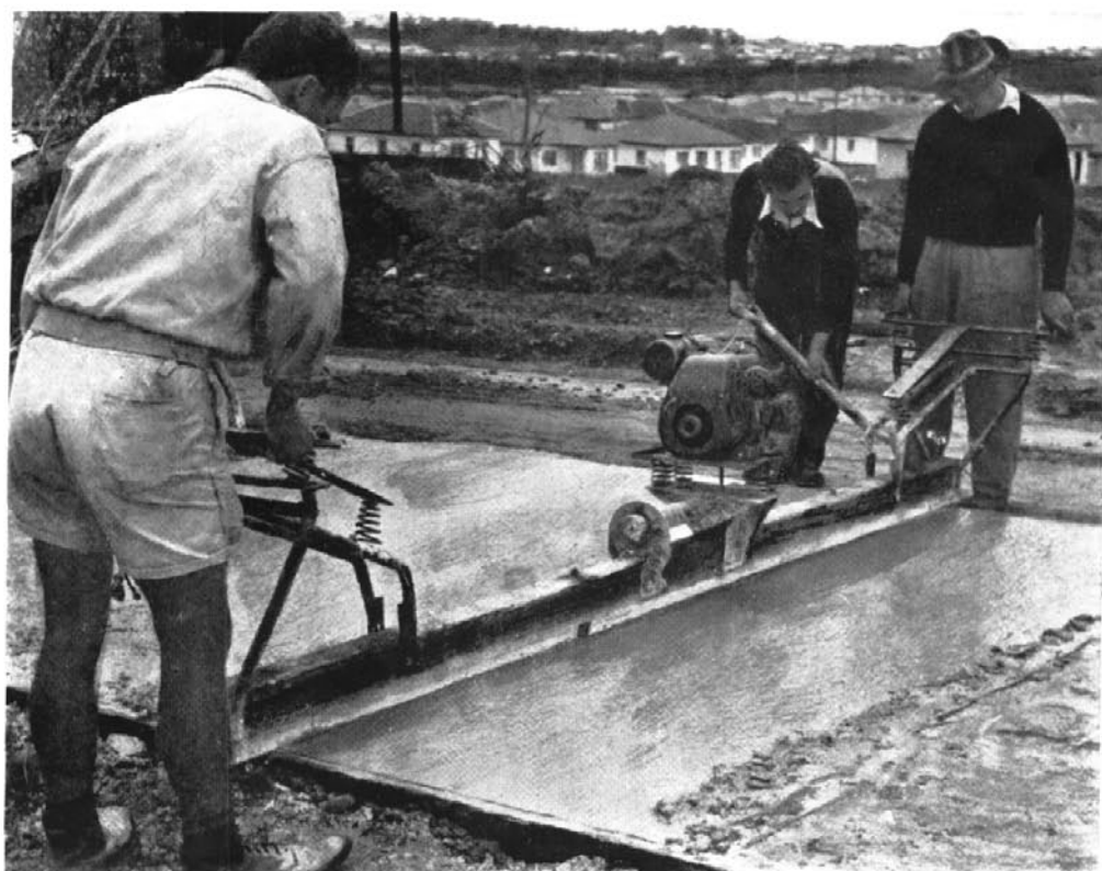
Tamping and screeding; Vibrator attached to Screed.
