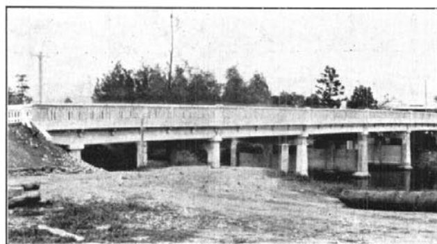
Concrete bridge, 210 ft. long, recently completed over the Brunswick River at Mullumbimby, North Coast Highway.
