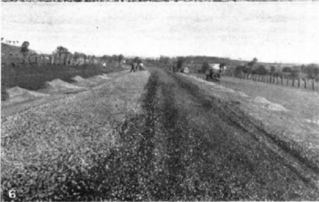
2. Mixed tar and slag in the first windrow.
