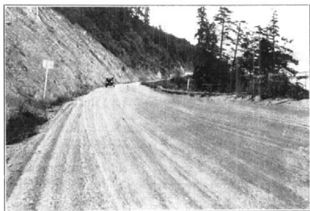
Fine crushed rock surfacing on the Pacific Highway, Washington, U.S.A.*
