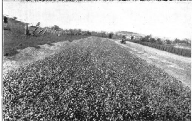
1. Slag spread, ready for spraying.
