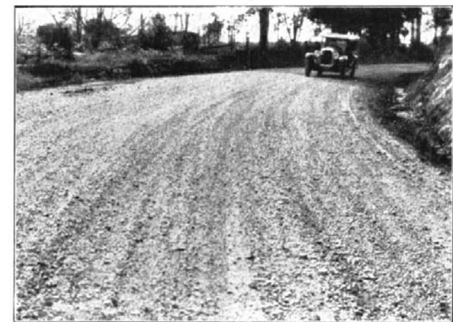
Fine crushed rock surfacing between Raleigh and Coff's Harbour, on the Pacific Highway in Bellingen Shire.
