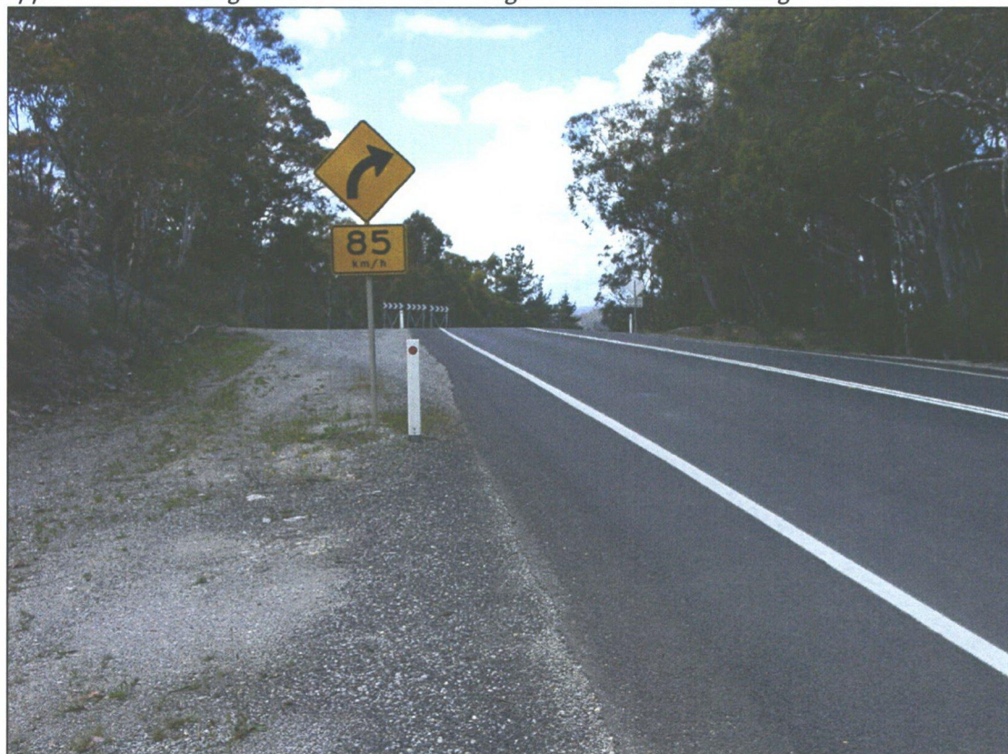
Photo 6: View south to section in the Highway known as the 'Capertee Crest' at approximate Chainage 650. Note the short sight distances for travelling vehicles.
