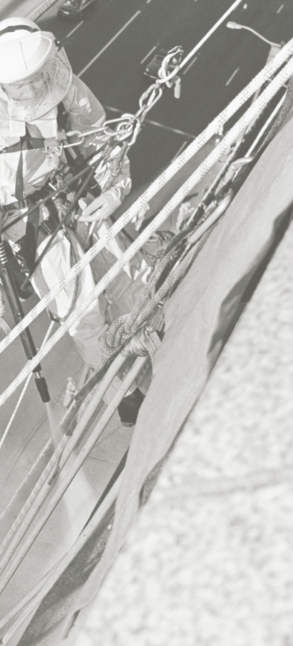
Sydney Harbour Bridge pylons are cleaned by abseiling RTA riggers.
