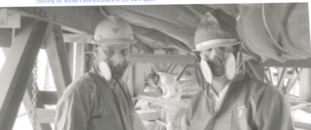
RTA removal of lead paint on McFarlanes Bridge, Maclean, required protective clothing for workers and enclosure of the work space
