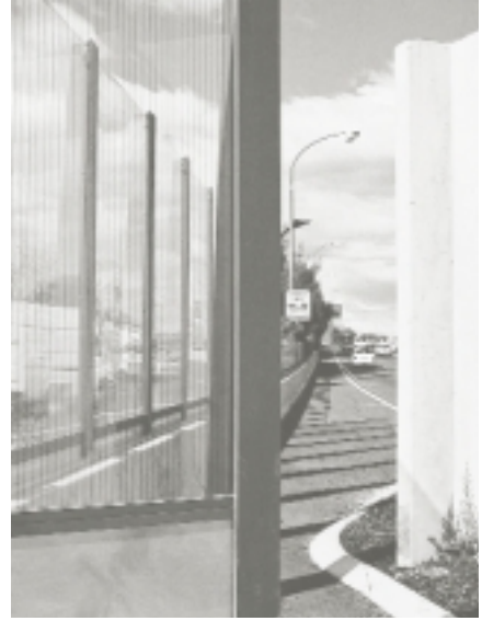
Innovative use of transparent acrylic noise walls on the Eastern Distributor
