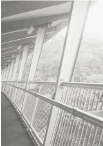
The Woronora Bridge's integrated 'bushland' boardwalk for pedestrians and cyclists
