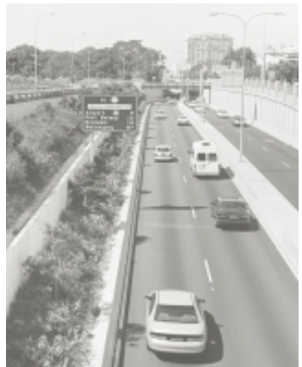
The Eastern Distributor achieved urban design excellence
