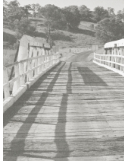
The RTA is restoring or replacing country timber bridges, which are vital for local families and businesses to access school, markets and services.
