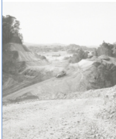
Yelgun to Chinderah is the largest road project underway in rural Australia
