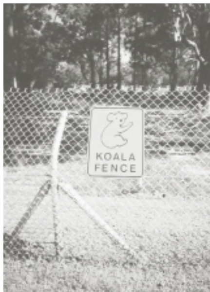
Koalas are unable to cross floppy top koala fences as the top bends back with their weight and prevents them from climbing over onto the road.
