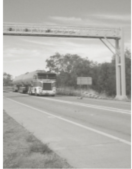
21 Safe-T-Cam sites monitor speed and fatigue of heavy vehicle drivers
