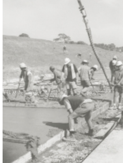
Workers lay M5 East Freeway pavement
