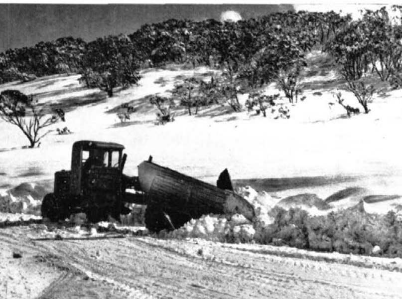
Snow removal on Mount Kosciusko Road using V-plough on motor grader
