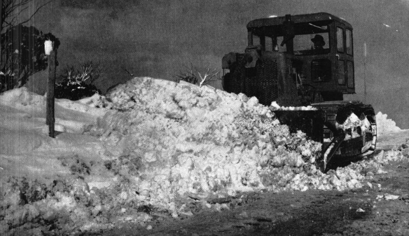
Snow clearing by dozer on Mount Kosciusko Road east of Smiggin Holes
