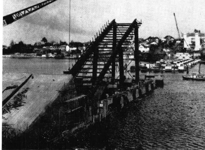
Falsework being erected
