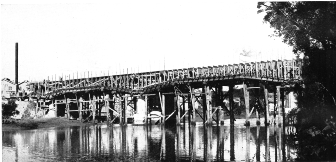
Falsework and Forms for a long-span continuous reinforced concrete girder bridge over a tidal stream, there being small risk of flood damage.
