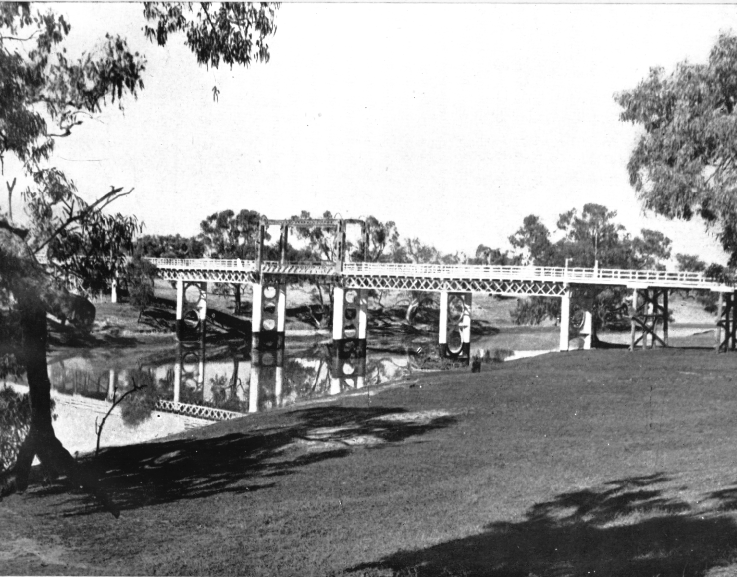
Bridge over the Darling River at Bourke.
