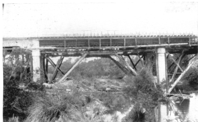
Falsework and Forms for a rigid frame reinforced concrete beam bridge over a stream subject to flooding. A substantial opening has been provided for flood flow. Two sets of longitudinal timbers have been used on account of haunches.
