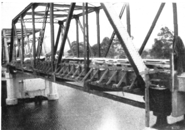
Frames and Forms for the kerbs of a truss span having a reinforced concrete deck.
