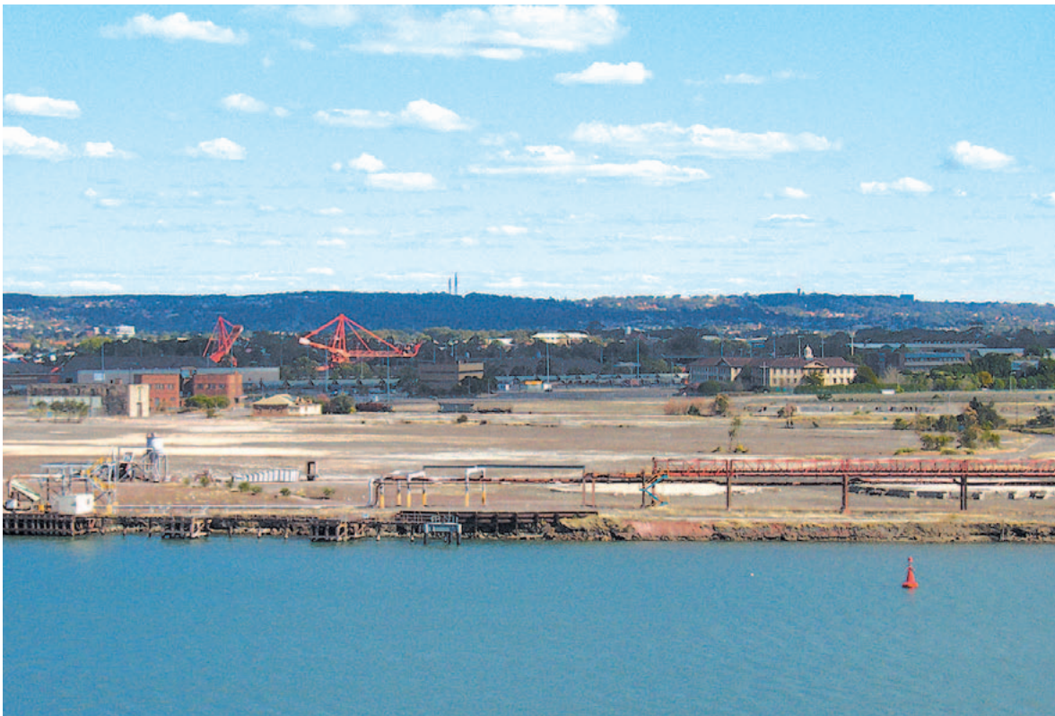
RLMC has developed a $110 million remediation strategy for its Mayfield site
