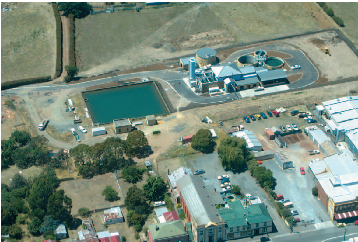
New water treatment plant at Langford, Tasmania
