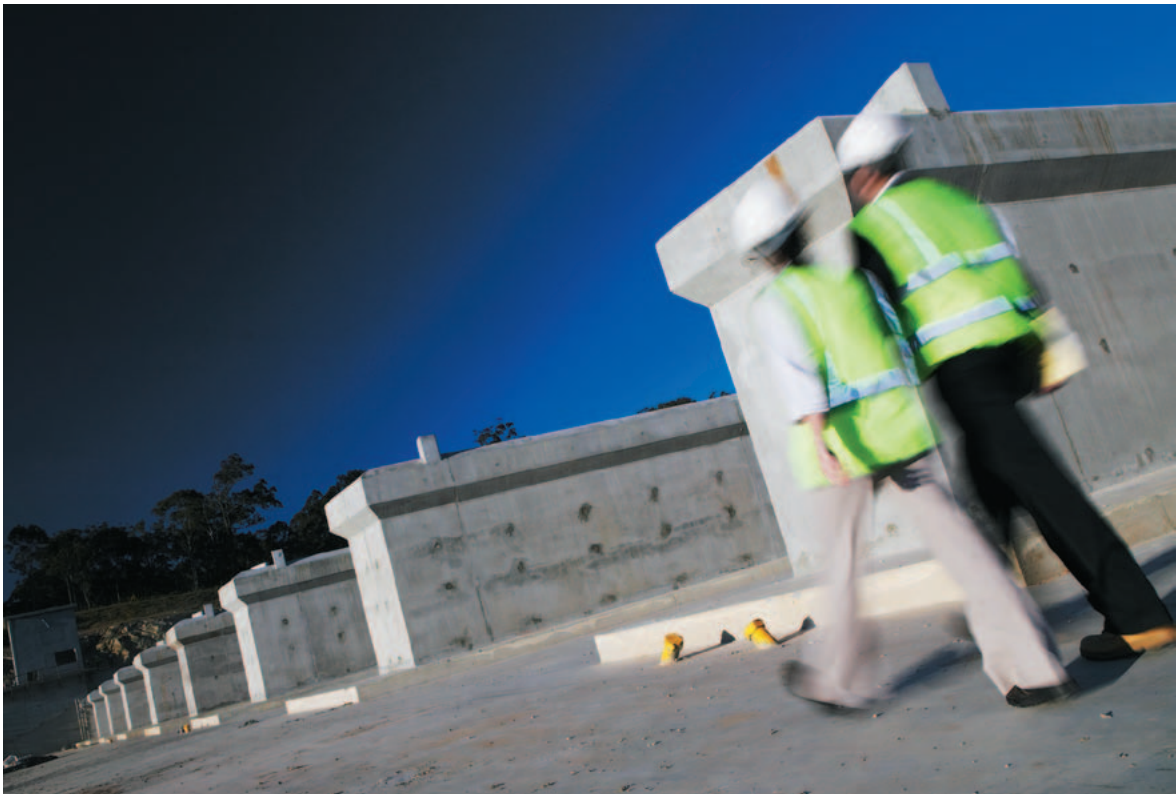
The new labyrinth spillway at Grahamstown Dam
