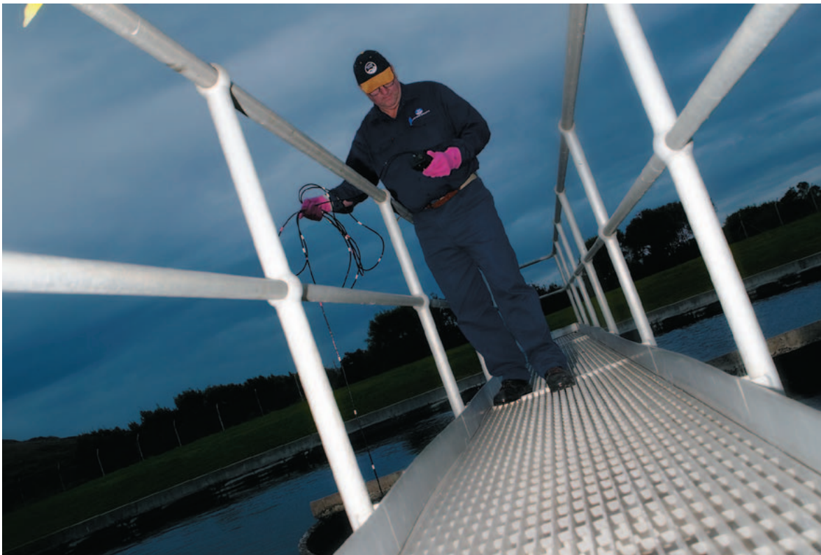
A suspended solids meter measures the level of mixed liquor suspended solids in clarifiers
