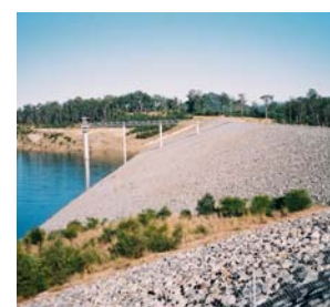
Cowarra Dam. Surveillance of this 40m high earthfill dam near Port Macquarie is at a high level during its initial filling phase.
