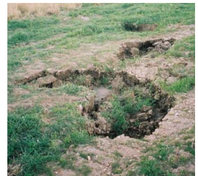
Warkworth Tailings Dam. Surveillance of this dam in the Hunter Valley detected an incipient piping incident in September 2003 with remedial actions quickly implemented by the owner.
