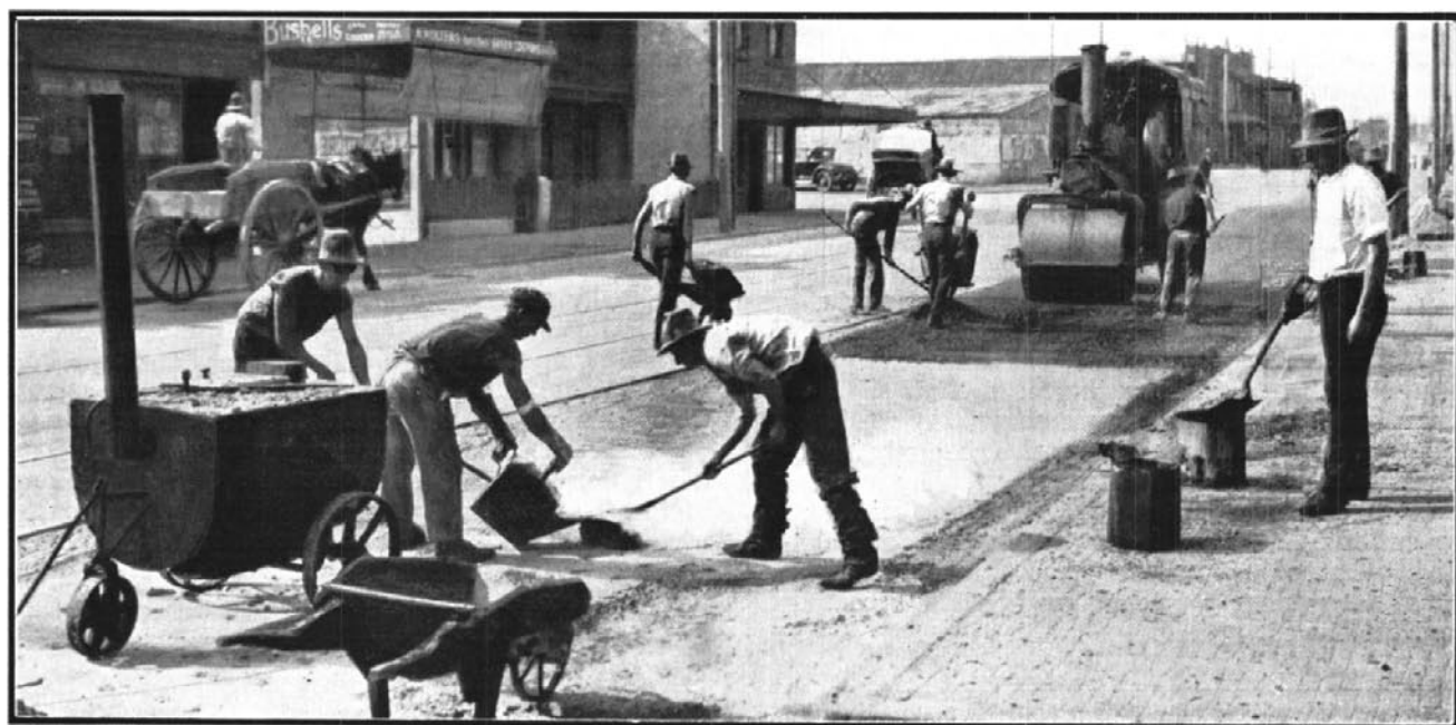
Application of bituminous surfacing to concrete pavement, Botany-road.
