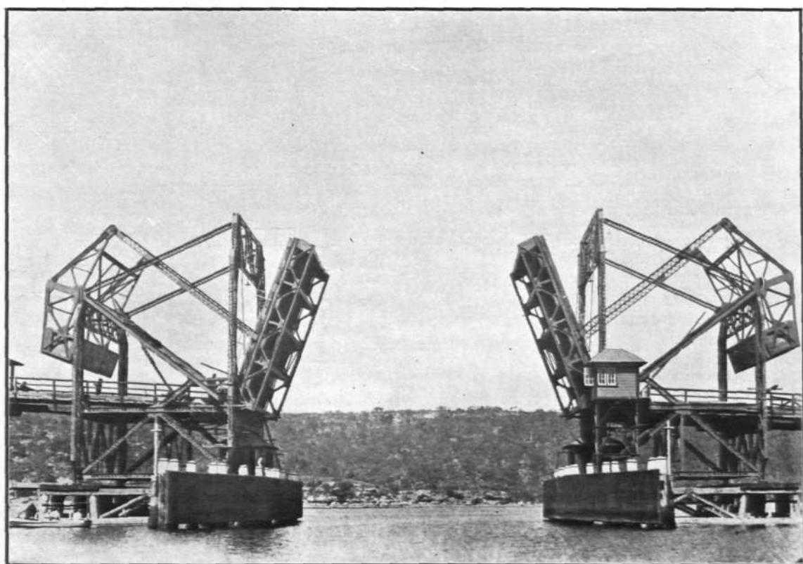
Open Bascule Span in temporary Timber Bridge at the Spit, Middle Harbour.
