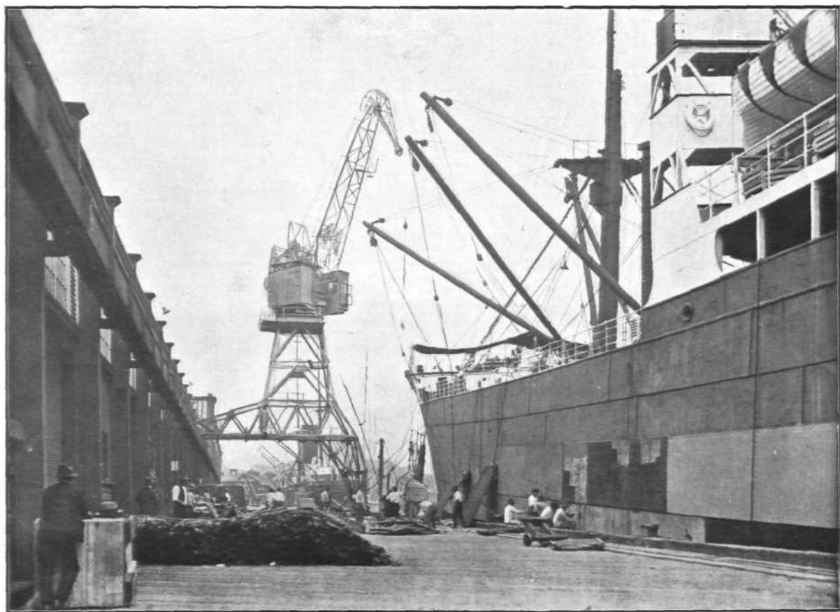
No. 1 Berth, Woolloomooloo, showing 2-ton Electric semi-portal Luffing Jib Crane.
