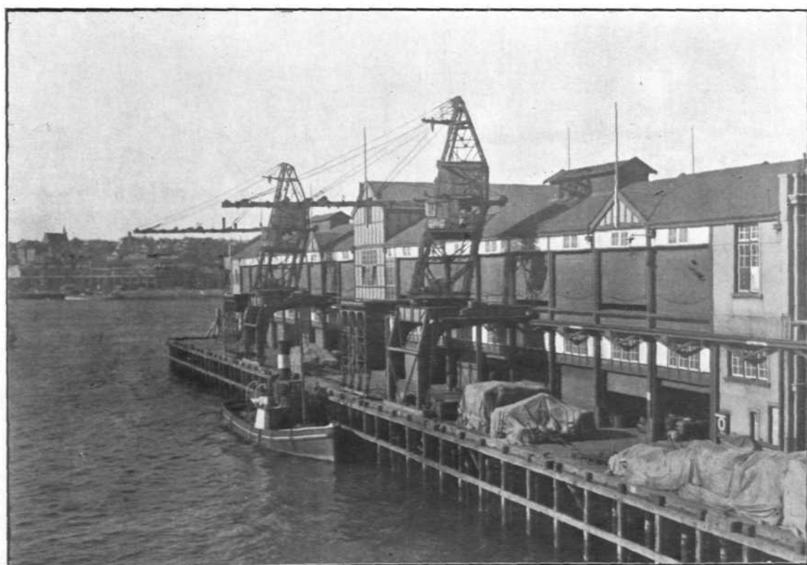
No 1 Berth, Walsh Bay, showing two 3-ton Electric travelling transporter Cranes and two travelling Gantries.
