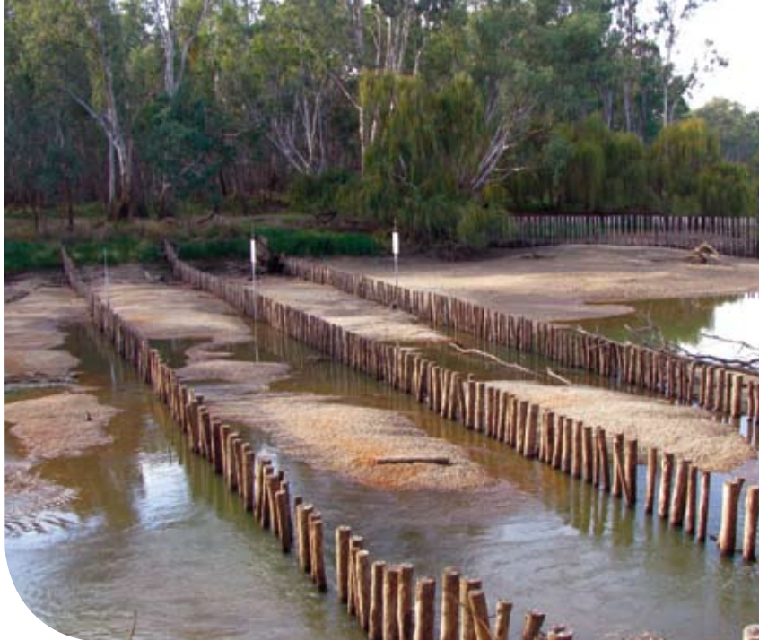
Full stream width pile fields at Boiling Downs Creek – expected to alter flows entering the anabranch
