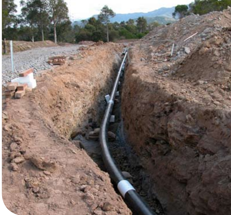
Top left: New gas pipeline for Colongra Gas Turbine project at Munmorah
