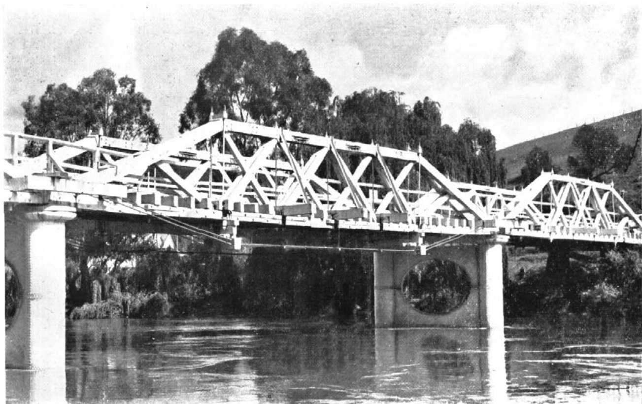
Undertrussing of span.
