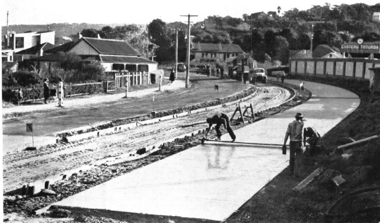
Concrete pavement construction in progress near Warringah Shire Council Chambers, Brookvale.
