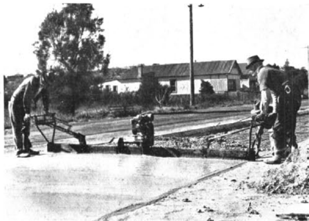
Vibrating screed at work.
