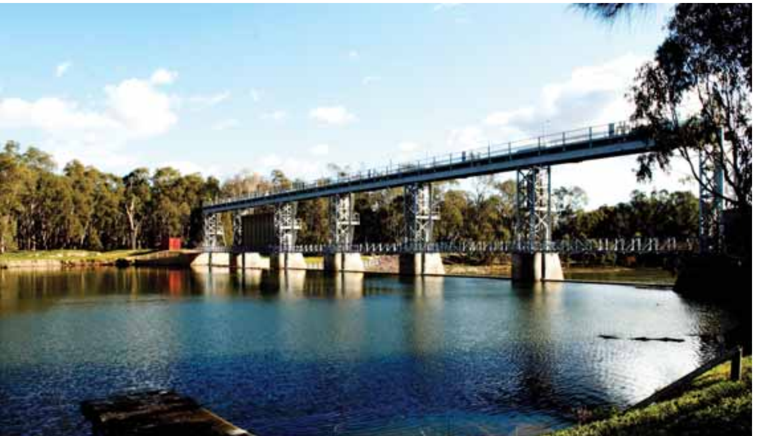
Gogeldrie Weir steel superstructure on the Murrumbidgee River near Leeton
