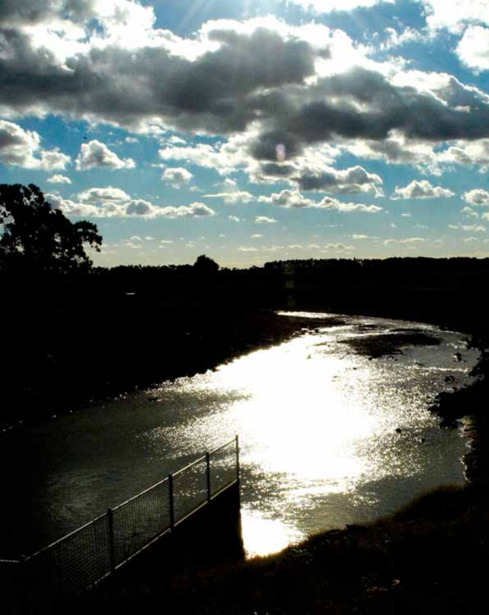
Gogeldrie Weir, near Leeton in the South Area, was one of the country locations visited by the State Water Board this year.
