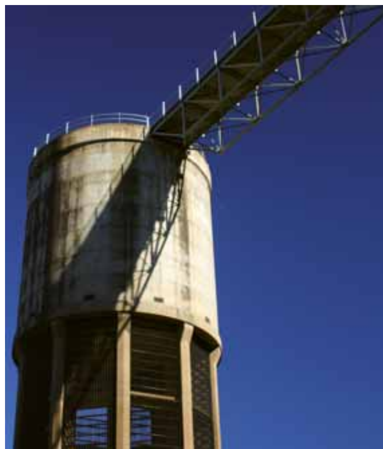
Intake tower at Burrendong Dam
