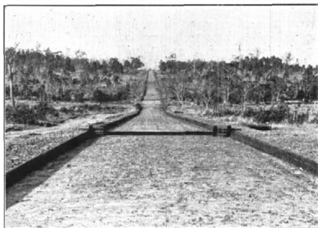
Road formed in readiness for construction of concrete pavement on Carne's Hill deviation, looking south.
