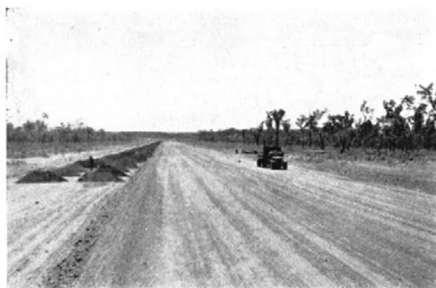
Fenton Aerodrome—Resheeting prior to sealing.
