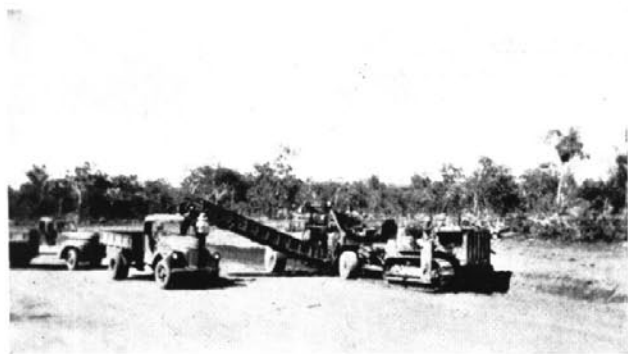
Elevating Grader loading gravel.
