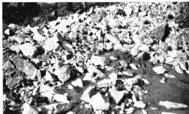
Mud welling up under displacement of filling.
