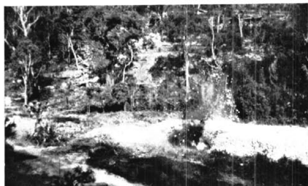
Side shots exploding surcharged fill. Extra height is about 2 feet 6 inches.
