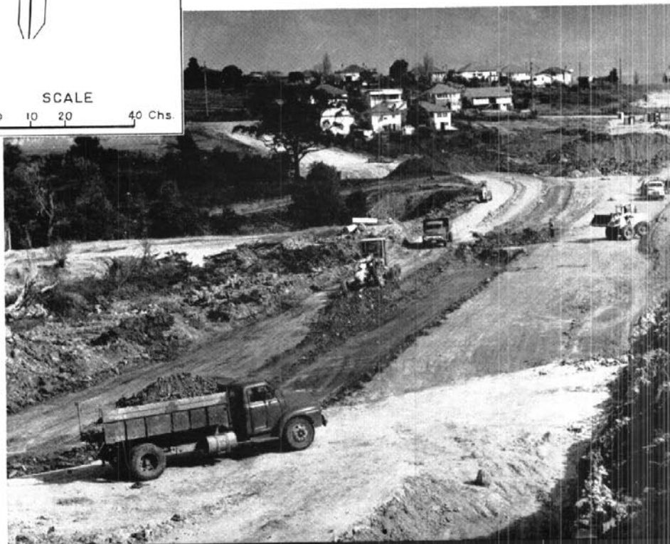
The Wollongong by-pass road under construction south Reserve Street
