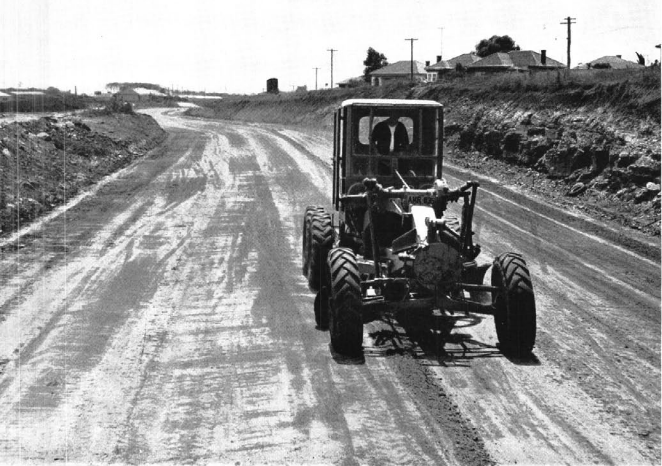
g of formation in progress on the by-pass road
