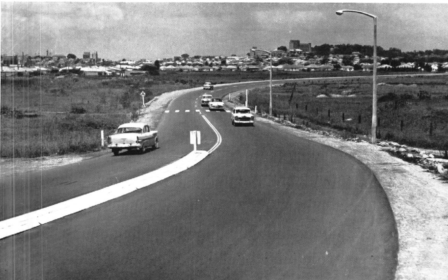
Completed section of the by-pass road near its junction with the Prince's Highway north of Wollongong
