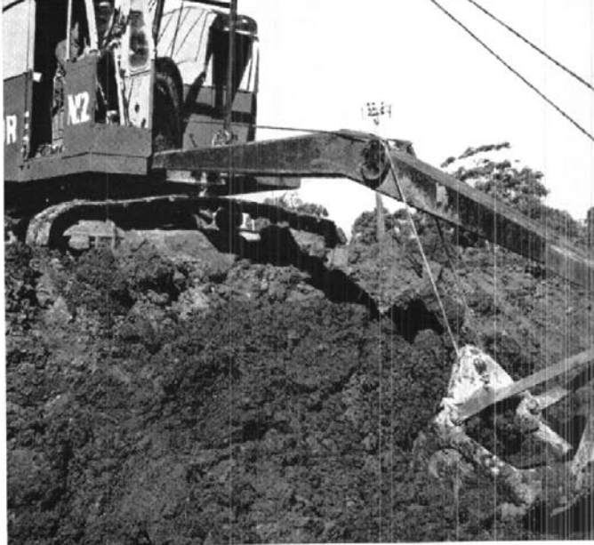
Excavation work on the Wollongong by-pass road
