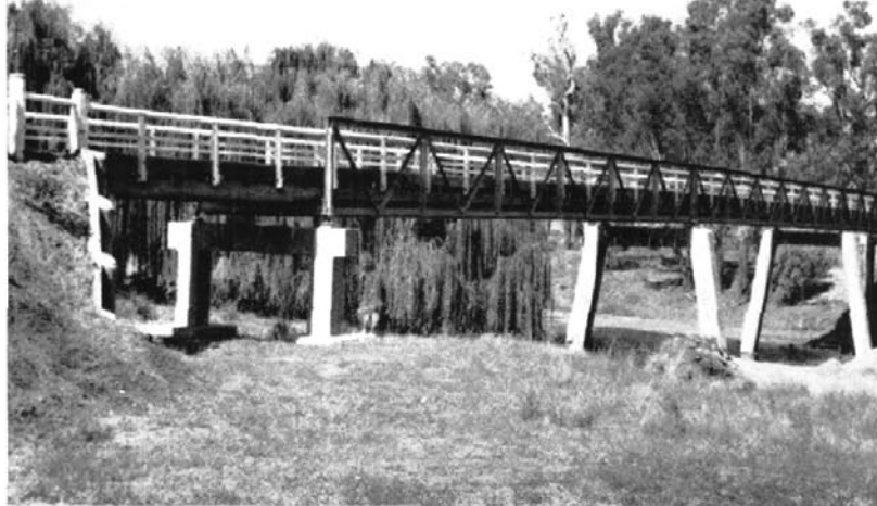
New bridge over the Namoi River, Harparary
