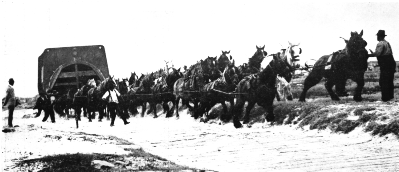
Hauling a 25-ton condenser section to Bunnerong Power Station in 1927.
