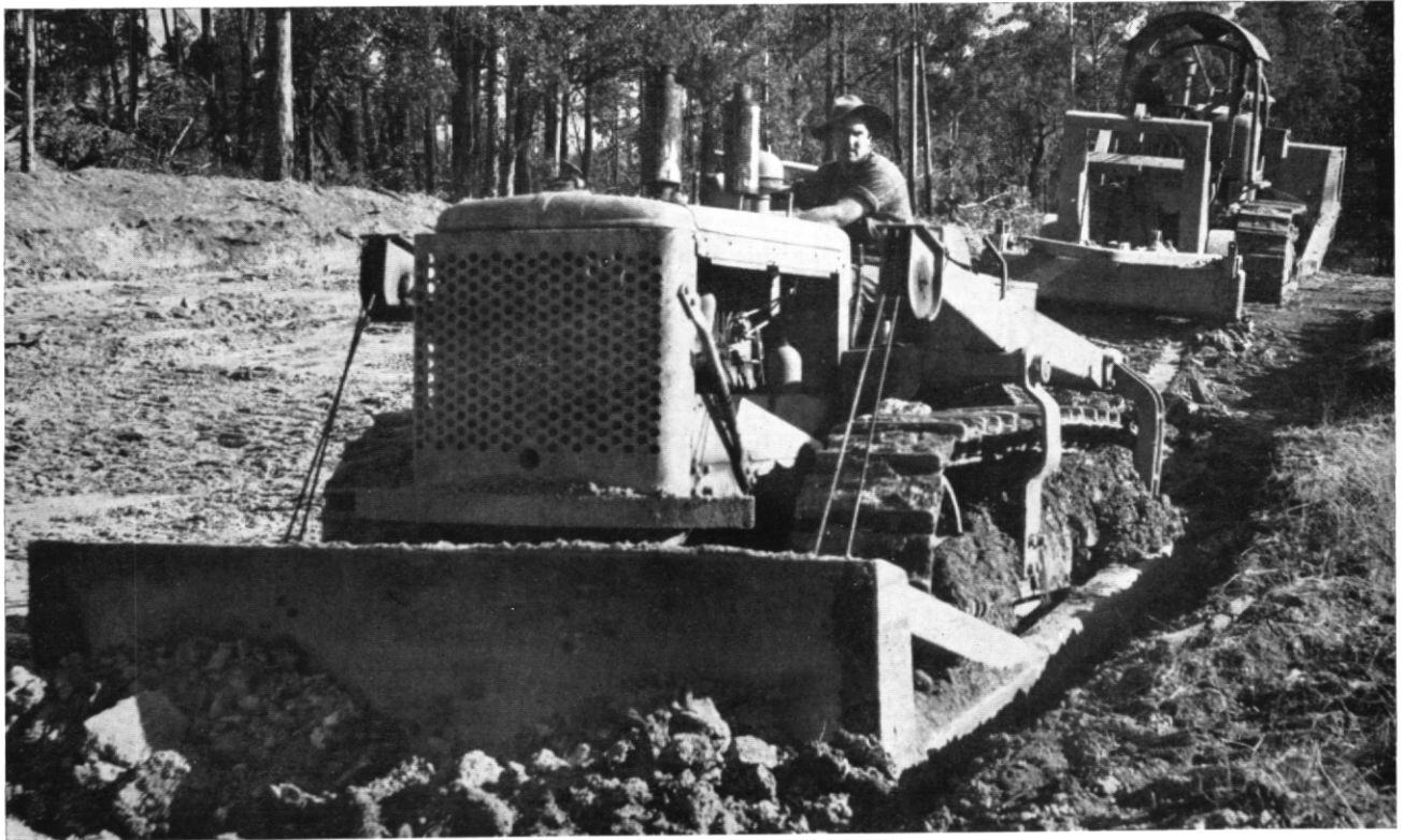
Excavation in progress near Nabiac.
