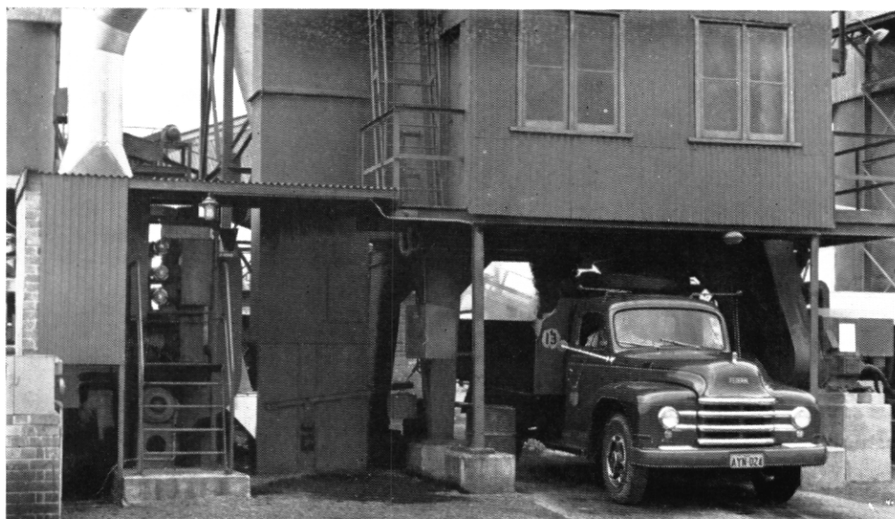
Delivering hot-mixed material to motor vehicles.
