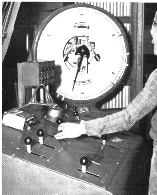
Control room for weigh batching.
