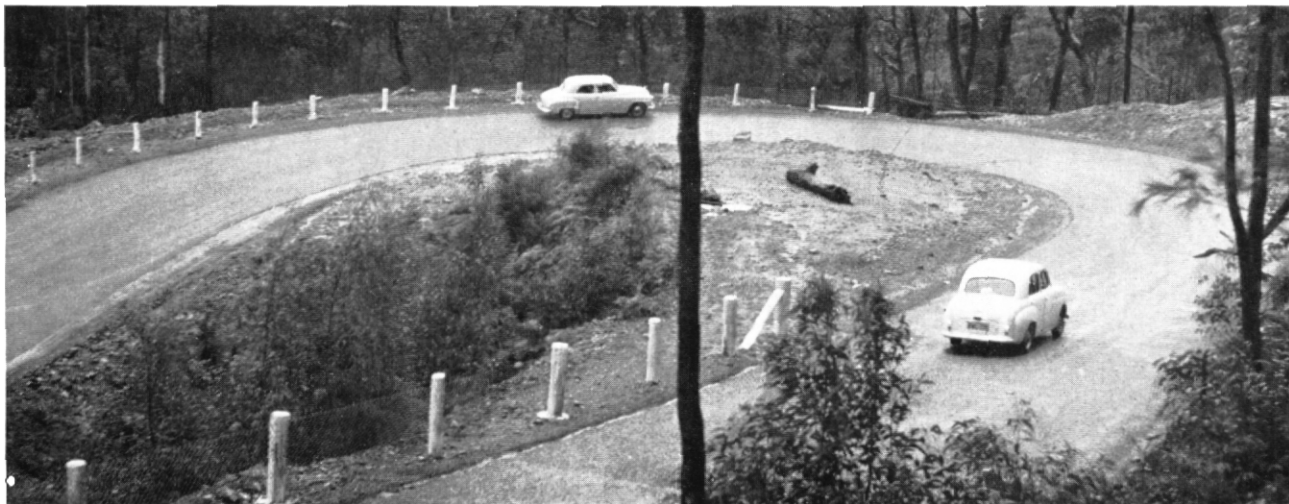
Improvement at Devil's Elbow between Bulahdelah and Booral on route being temporarily used by Pacific Highway traffic.
