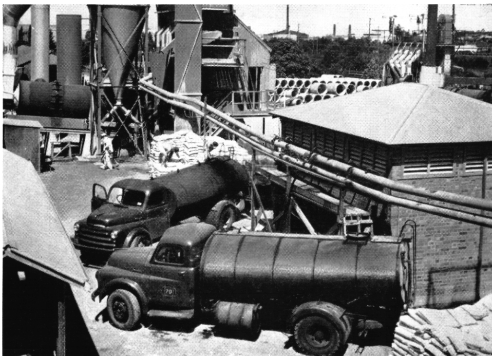
Unloading bitumen from road tankers to storage and heating unit.
