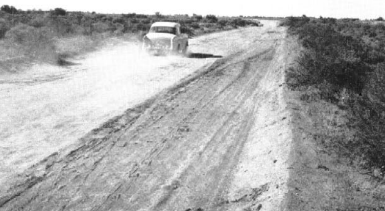
The Silver City Highway south of Broken Hill prior to reconstruction and bitumen surfacing
