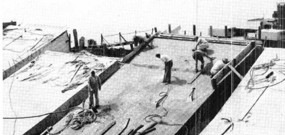
The arch thrust blocks nearing completion on the Gladesville side
