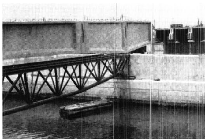
Cantilever beam in the northern approach span of the new bridge showing launching truss
