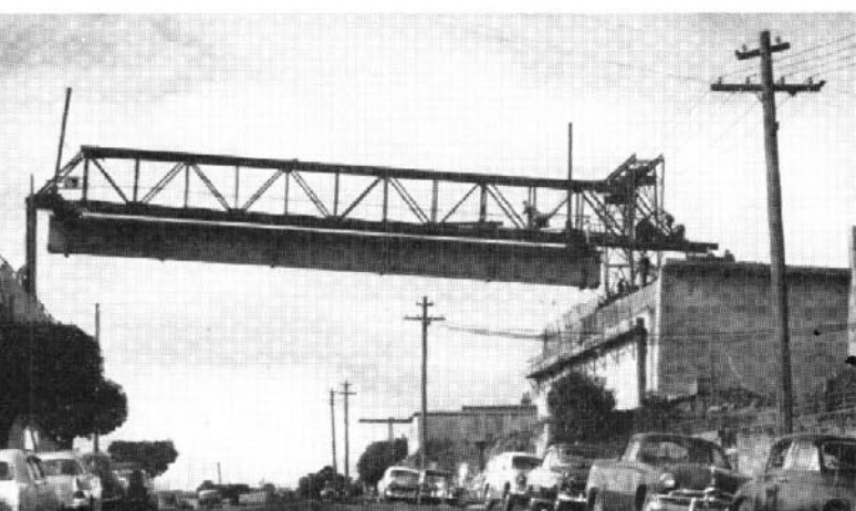
Launching a deck beam for an approach span
