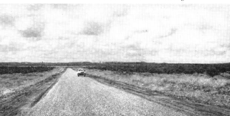
The Silver City Highway south of Broken Hill following reconstruction and bitumen surfacing
