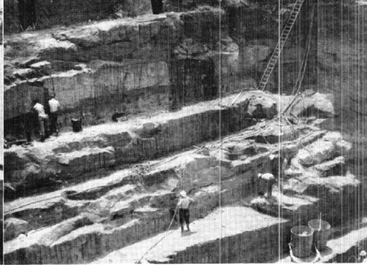
Left:—Construction of coffer dam on the Drummoyne side of the river
