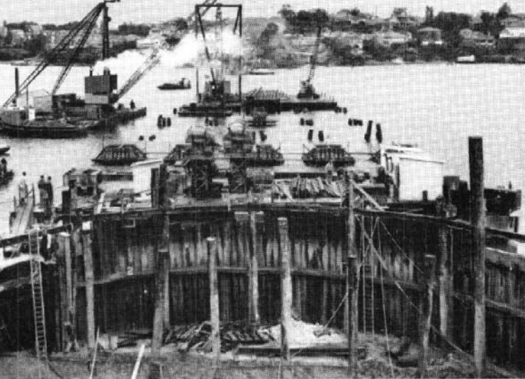
Left:—Construction of coffer dam on the Drummoyne side of the river
