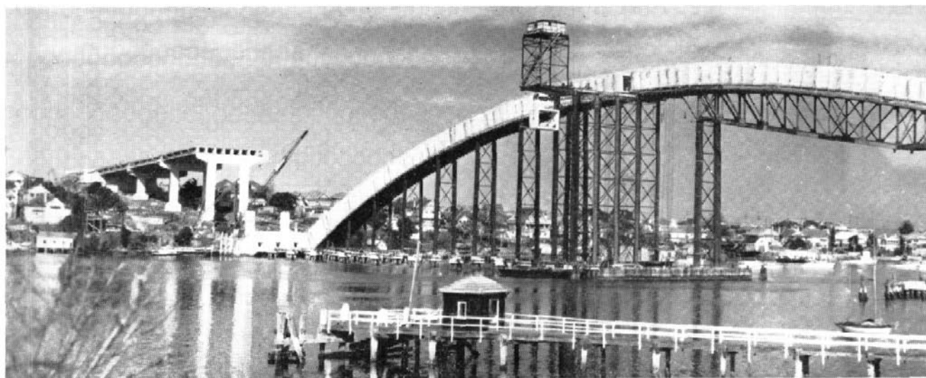
The last concrete block for the first rib of the arch being hoisted to the top of the falsework
