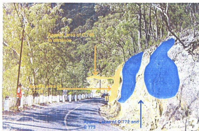
C7.58- view south towards cut section
