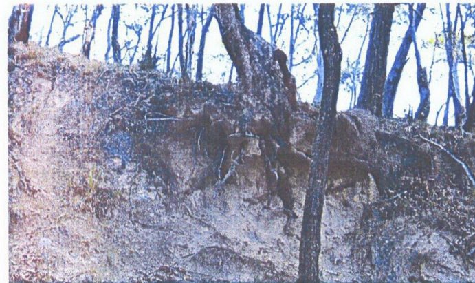
Access track- view north west- under mined tree
