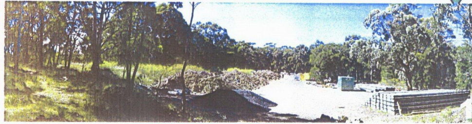
RTA Storage Compound- view south
