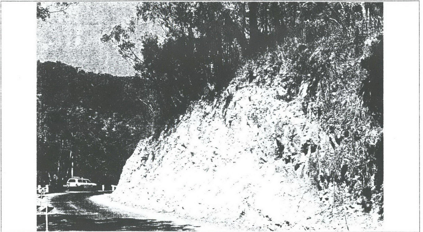
Photo 1: Extent of completed works at Walls 40/41.
