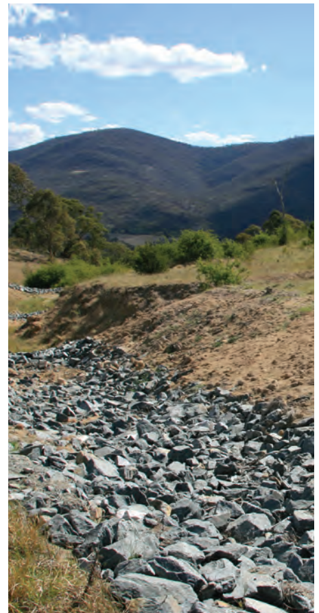
A rock chute was constructed to address severe gully erosion problems
