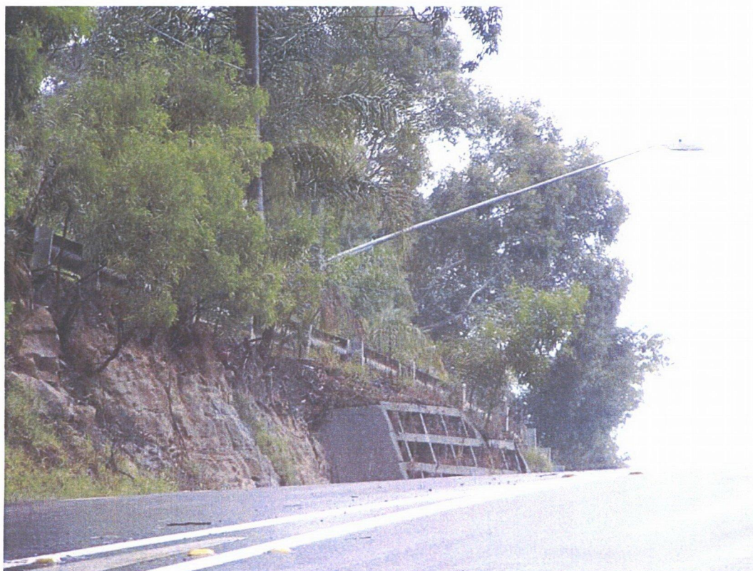
Figure 5.3 - Road cutting on the eastern side of Avoca Drive. Original soils have been excavated and removed from this area.
