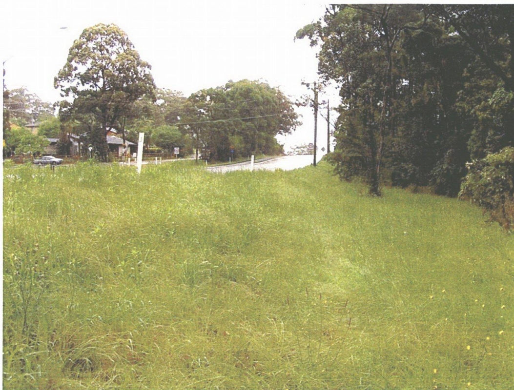
Figure 5.2 - Fill on western side of Avoca Drive. Original ground has been covered by more than 2 metres of fill.
