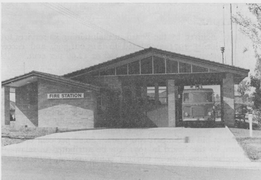
Blacktown Fire Station
