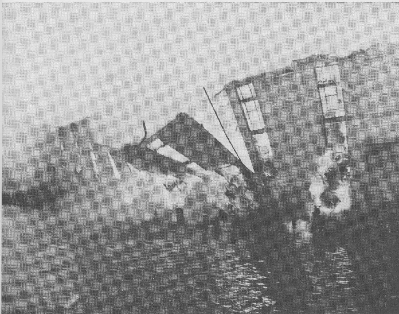
Wall collapse during extensive fire at premises of John Fairfax & Sons—Pymont
