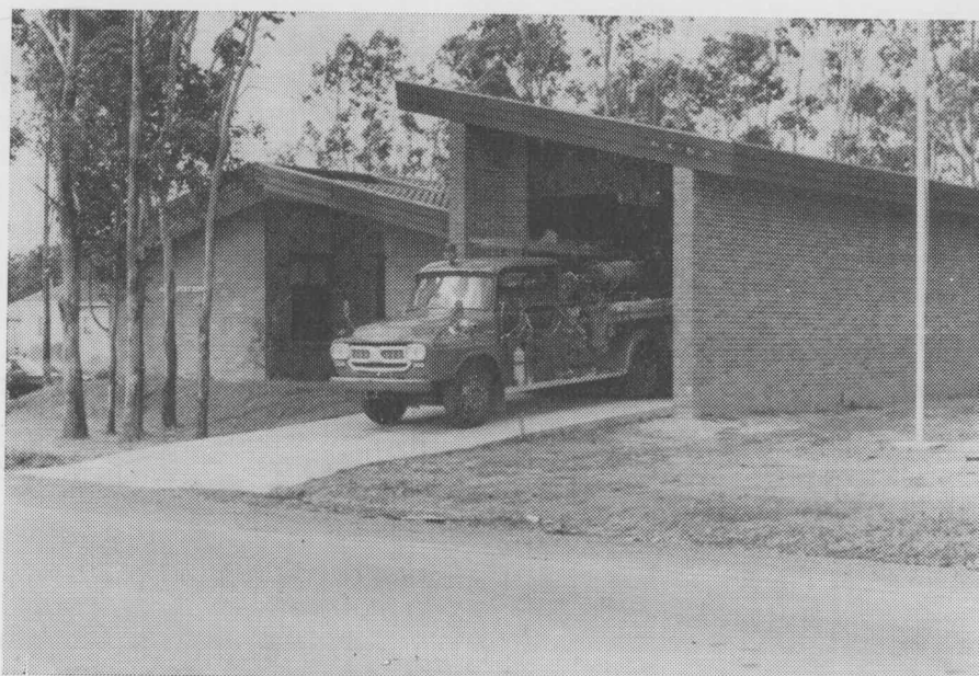
Mt Druitt Fire Station
