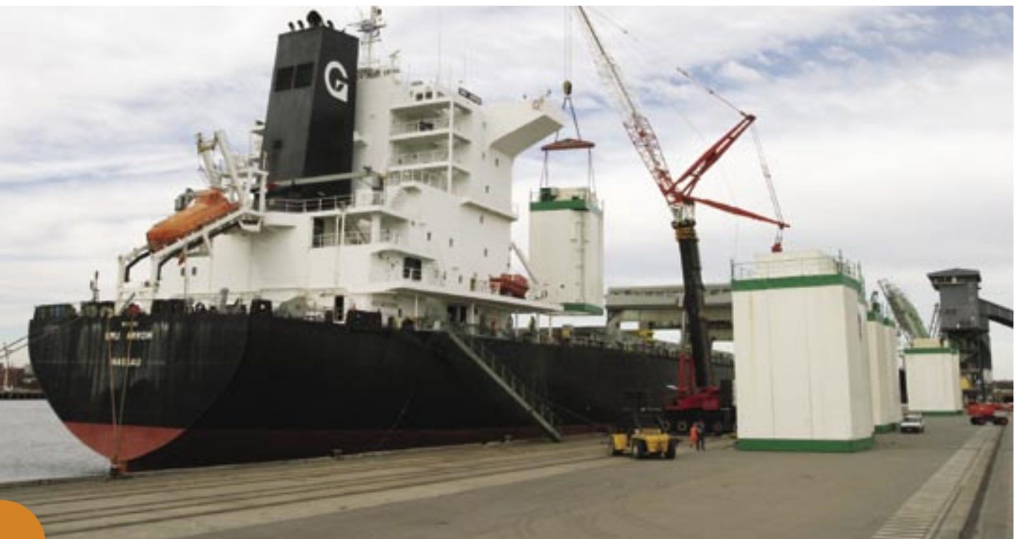
Frozen orange juice storage tanks are unloaded for installation at the new receiveal facility.
