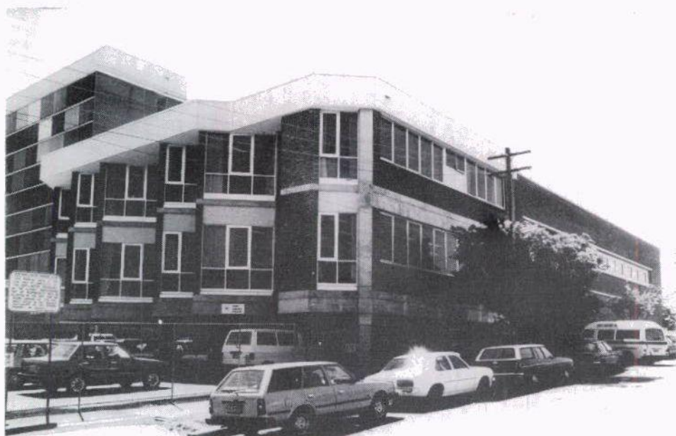
The Traffic Authority of New South Wales' new headquarters at Rosebery.
