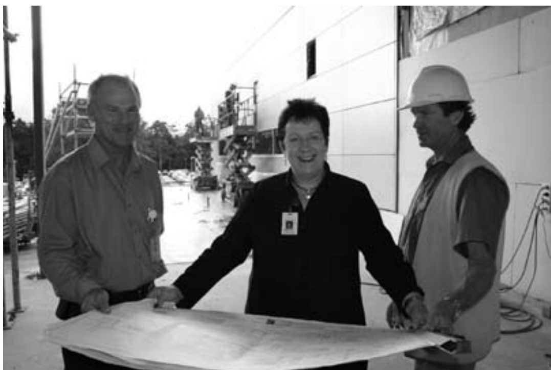
Inspecting the plans on the construction site of the Cardiac Catheterisation Laboratory is the General Manager of Coffs Harbour Health Campus, Margaret Bennett, Assistant Maintenance Manager, Ian Dellar, and Kevin Hartley, the foreman for builders, F.M. Glenn.
