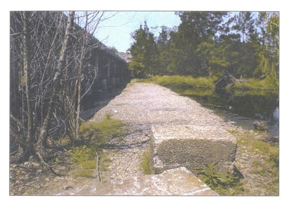
**Plate 3**: View of existing temporary weir constructed (by RTA 2000) along the southwest section of the existing bridge across the associated flood channels. The photo also includes one of the concrete blocks scattered across the main channel, placed during extraction activities.
