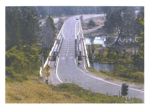
**Plate I**: View of Yarramundi Bridge / Springwood Road across the Nepean River, facing west. The Proposed new bridge would be 4m edge to edge downstream of the existing bridge with minor road re-alignments.
