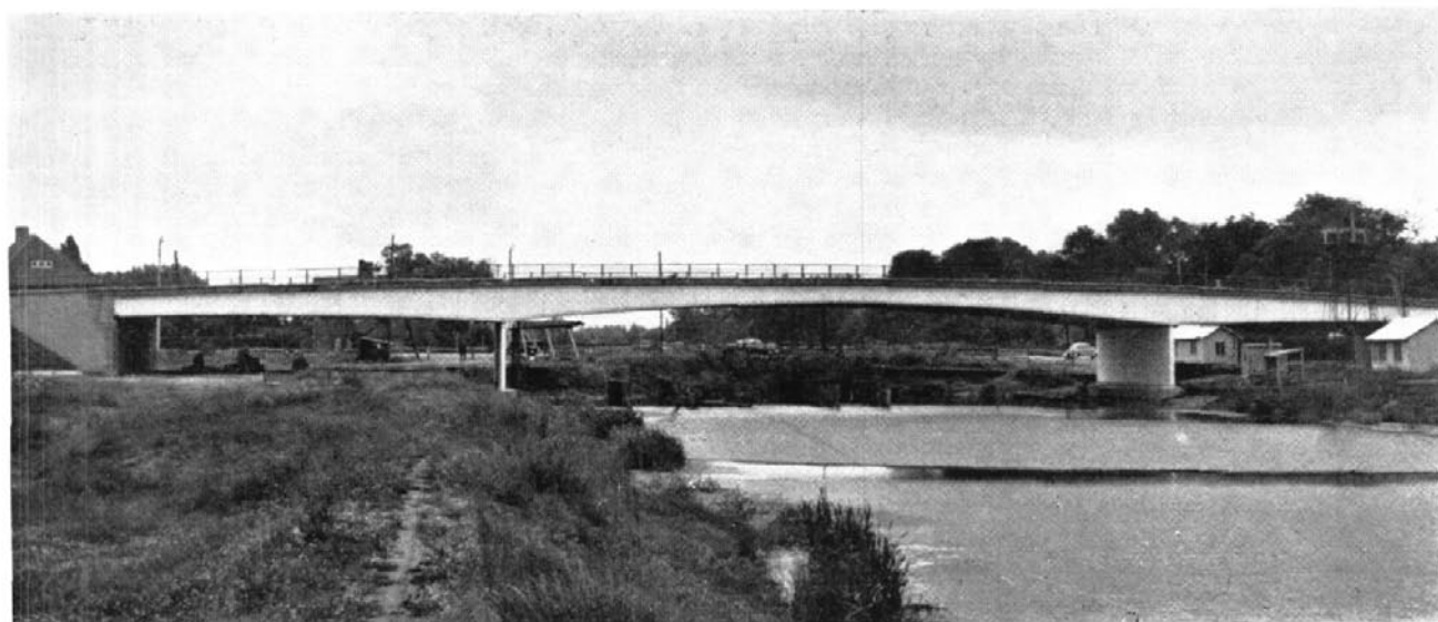
Ring Canal Bridge at Ghent, Belgium. Side view of structure. Note thin diaphragm piers which are hinged at bottom, all expansion being at one abutment, the other being fixed.
