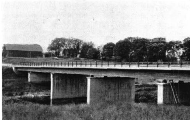
Bridge on Sagan via Östanbro near Enköping, Sweden. 5 span continuous girder R.C. Bridge using high tensile reinforcing bars.
