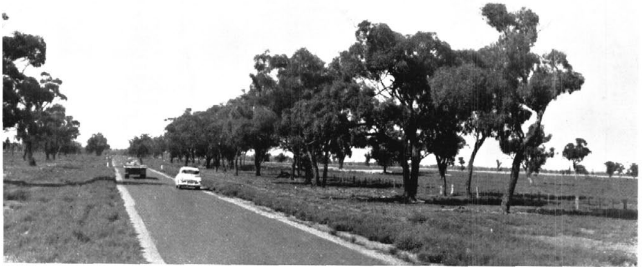
View of recently completed work on State Highway No. 21 in the Shire of Murray.
