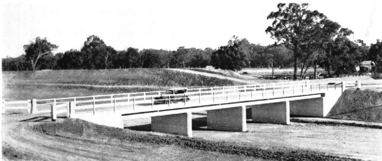
A concrete crossing over the main canal which supplies water to the Berriquin and Wakool Districts.
