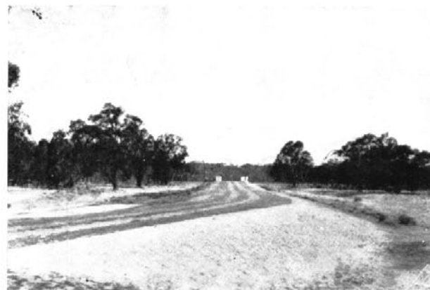
New construction Developmental Road No. 1146.
