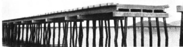
Sand Point Bridge, Lake Pend, Oreille, Idaho, U.S.A. Section of work showing precast spans in place.
