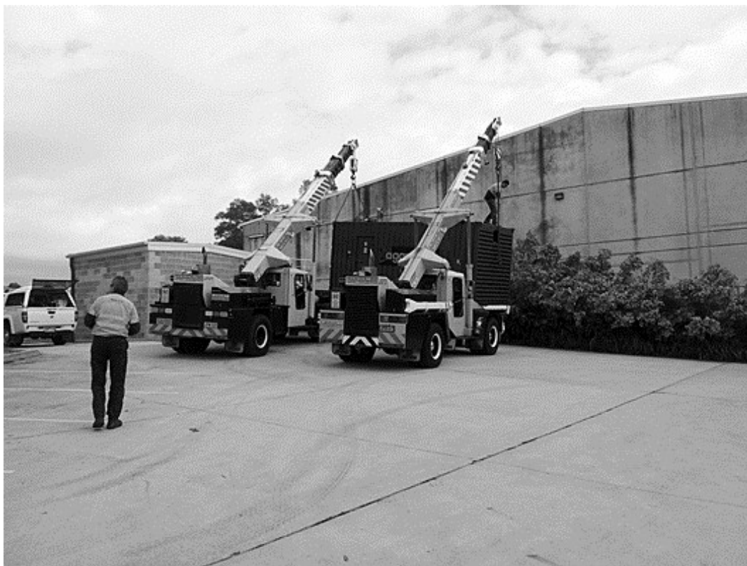
Generators being pre-positioned at Kingswood on 17/11/2012 in preparation for power shut down and electrical upgrade
