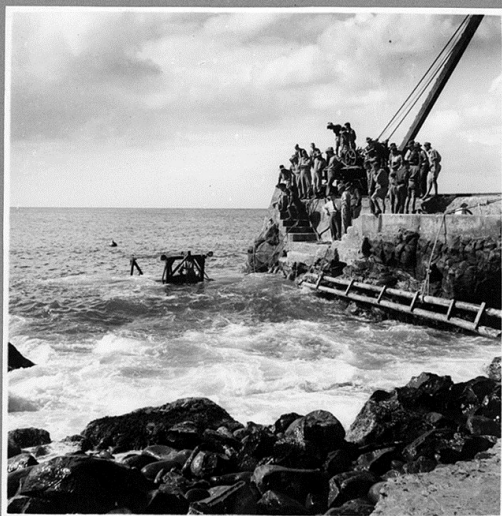
D8 Caterpillar Tractor in sea at Cascade. Slipped from barge (when not under D.M.R. control) in heavy surge.
