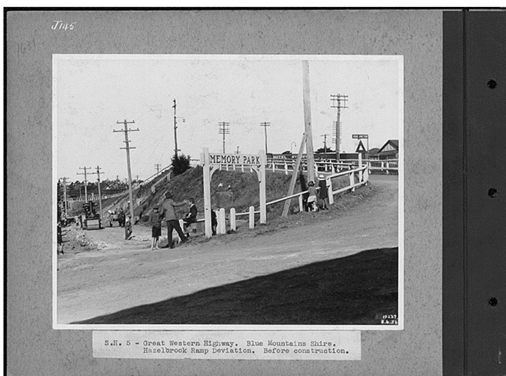
J145 -0 S.R.5 State Road 5—Great Western Highway. Blue Mountains Shire. Hazelbrook Ramp Deviation. Before construction. Digital ID: 20224_a038_001539
