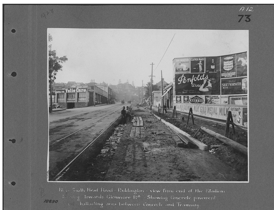
A12—New South Head Road—Paddington _ view from end of the Stadium looking towards Glenmore Road. Showing concrete pavement ballasting area between concrete and Tramway.
